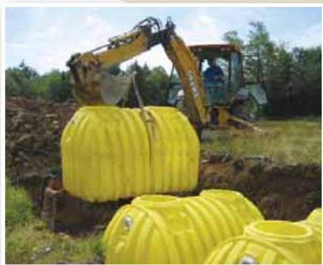
Figure 4. Penn State Environmental Engineering graduate student, Jessica Grembi, guides one of the pilot reactors into position at the Klondike-1 site.
