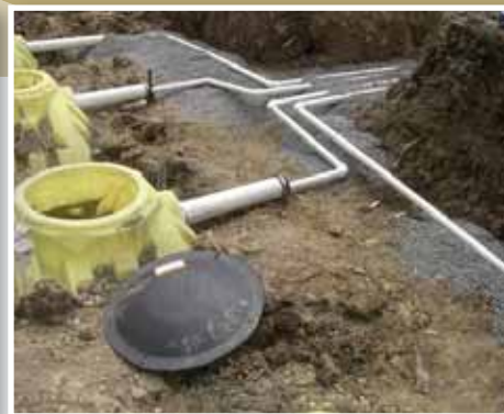
Figure 6. Influent to each of the reactors is provided through individual pipelines from the current primary oxidation/settling pond on site. After installation, the pipes were buried to prevent freezing in winter.
