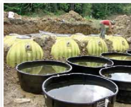
Figure 7. Effluent from each reactor will cascade into a series of two aeration/settling ponds, and then be piped to the existing aerobic wetland on site.
