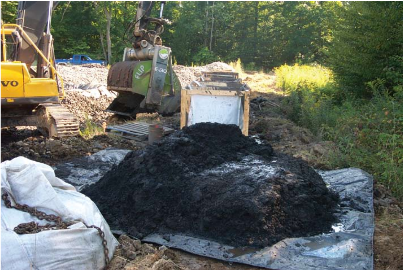
Figure 4. View of recovered manganese material excavated from wash pit.
