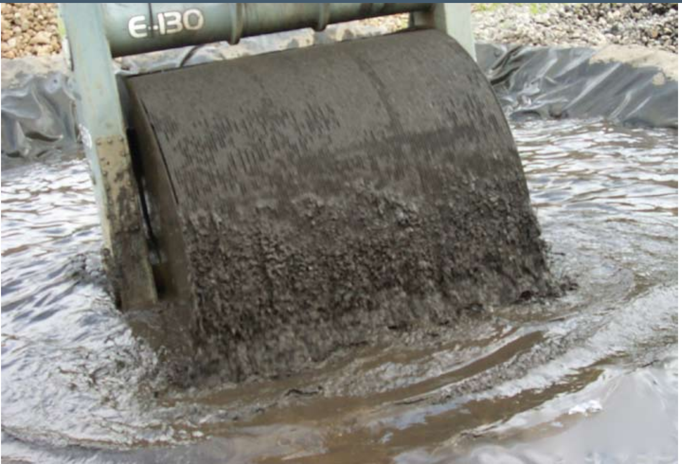
Figure 3. Close up of FlipScreen during manganese recovery operation.
