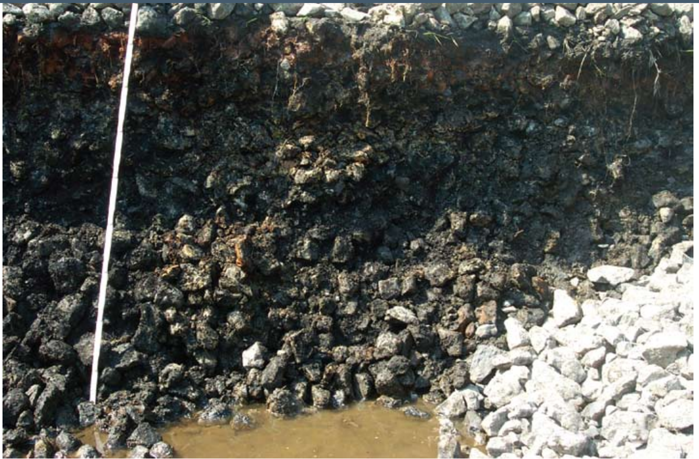
Figure 1. Manganese material filled the void spaces and coated limestone aggregate prior to recovery.
