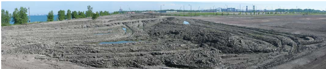
Picture 5. Slag field in June of 2004 covered with mud in various stages of drying. Mud was initially placed about a foot deep and bulldozed into piles as high as eight feet as it dried, making room for later placement.
