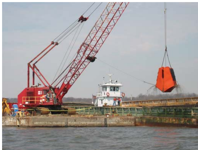
Picture 2. A crane excavates high solids mud from the bottom of the Illinois River near Peoria, IL. The sediment is as much as 25 feet thick in this area. It is placed in a standard 1500-ton hopper barge for shipment to Chicago.
