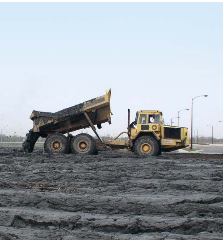
Picture 4. High solids mud being end-dumped on the slag field. The consistency obviated the need for a containment berm.
