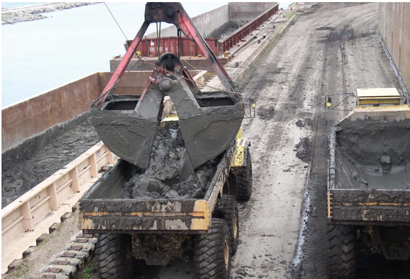
Picture 3. After a 168-mile river journey, the barges were unloaded to mining trucks in Chicago. Note the low water content of the mud.
