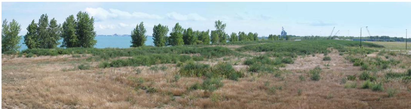
Picture 6. The former slag field supports vigorous vegetation in September 2005 one year after dredging. During the prior fall it was graded with a dozer to a depth of approximately 2.5 feet and seeded with grass.
