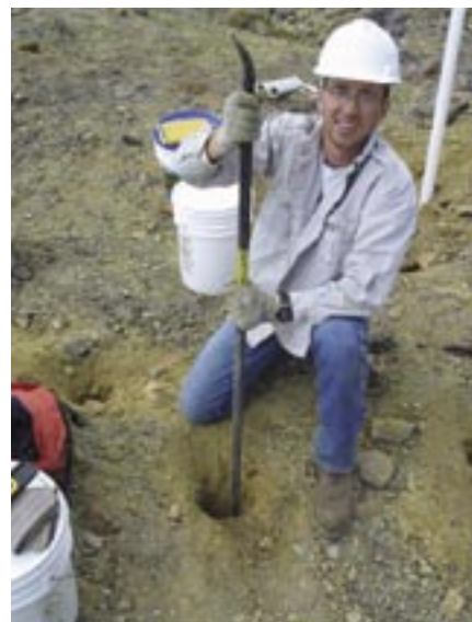
Fig. 4: Digging to install a tensiometer. One is already installed at the back.
