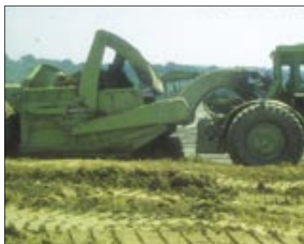
Photo 1. Scraper-pan replacing subsoil.
