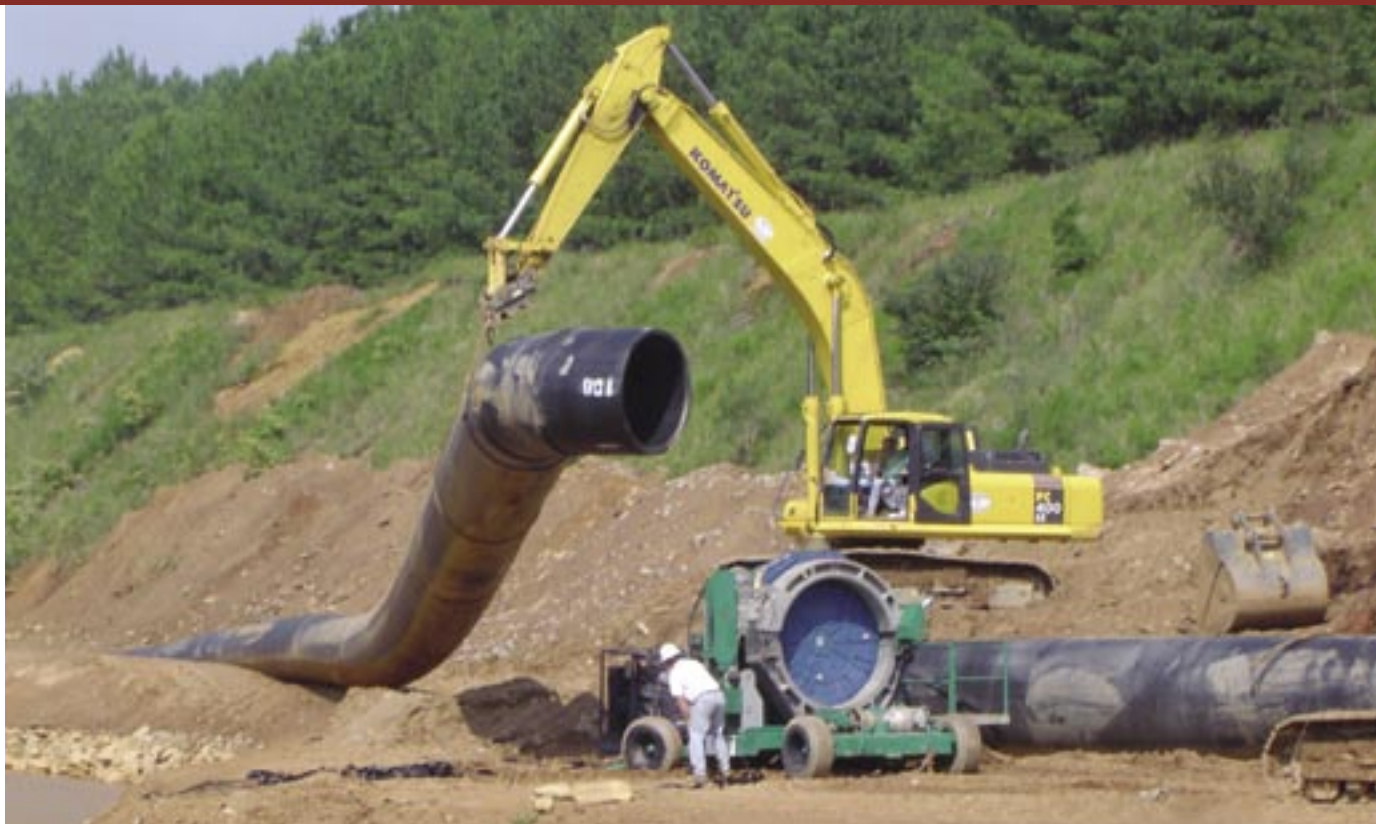
Picture 6: A pipeline of 3,000 feet made up of 63-inch diameter pipe was a construction challenge.
