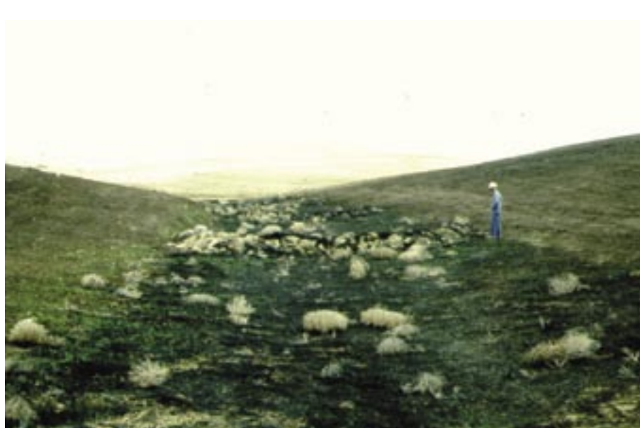
Picture 4: Rock check structures are installed in drainage channels to slow the water and allow sediments to fall.
