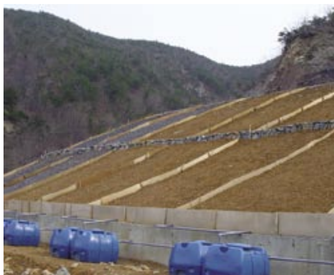
Picture 4: Application of amendments and installation of water collection tanks were completed and the plots were hydroseeded in May.
