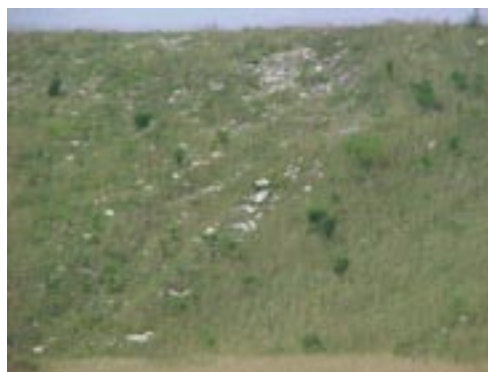
Some slopes were less compacted and were only rough graded.
