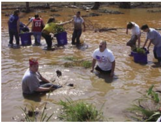
About 125 teenage volunteers helped the SRWC to plant the constructed wetlands at the Erico Bridge passive treatment system with guidance and an educational program provided by Aquascape Wetland and Environmental Services.
