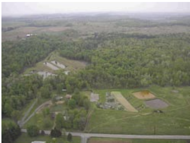
Passive treatment systems, such as the De Sale Phase 1 (bottom right) and Phase II (top left) that were designed by BioMost, Inc. and WOPEC, have significantly improved the water quality at Seaton Creek, the most heavily impacted tributary in the headwaters.
