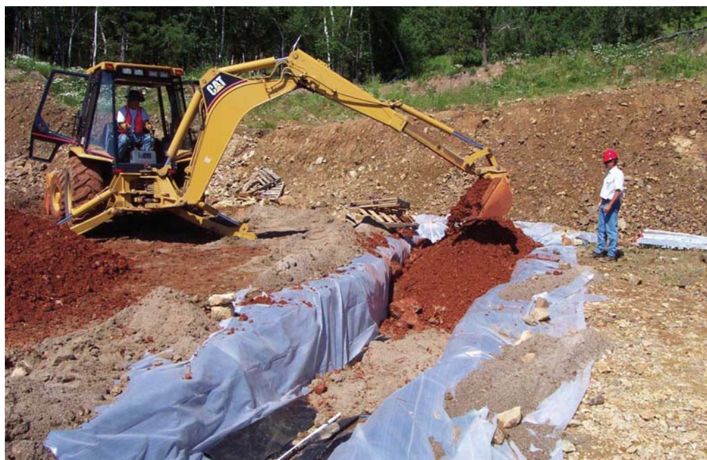
Filling trench with ViroMine™ waste rock mixture and filled trench
