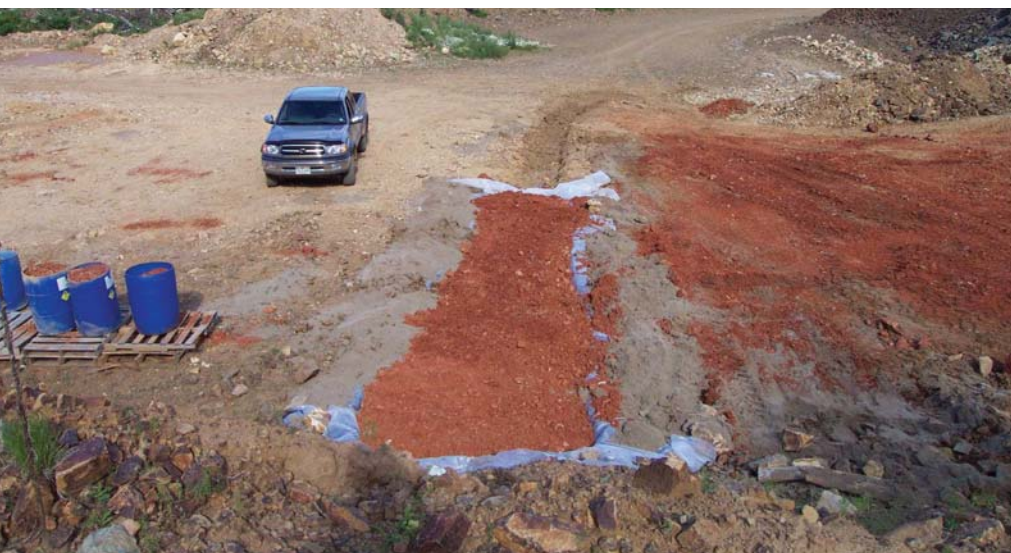
Filling trench with ViroMine™ waste rock mixture and filled trench
