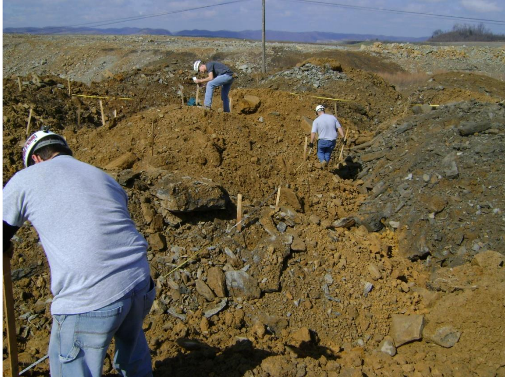
Figure 3. The 0.3-ha experimental area of brown sandstone and topsoil at Nicholas was constructed in 2009 and simply end-dumped with trucks. No leveling was done.
