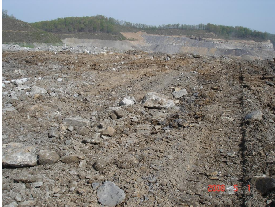
Figure 1. The 1-ha experimental site was constructed with mixed sandstone substrate, end-dumped with trucks, and the piles were flattened by one or two passes of a bulldozer.
