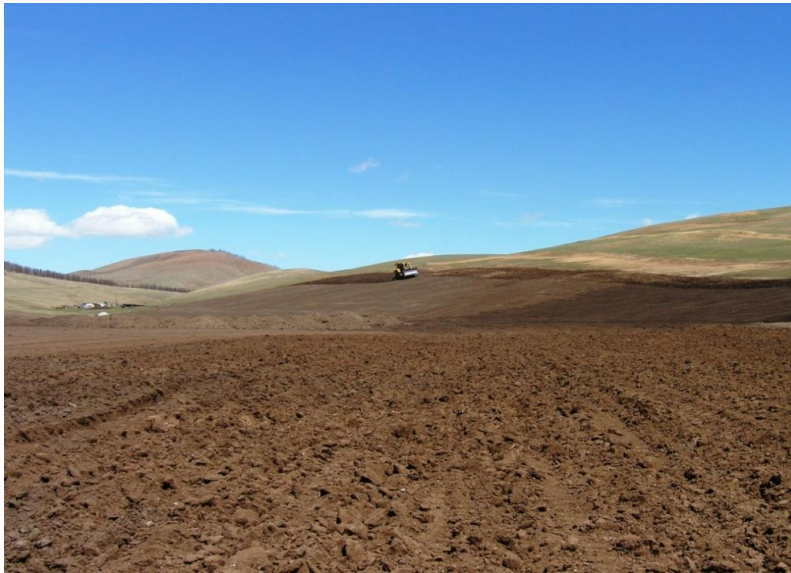
Figure 6. All areas were deep ripped on the contour. Note smooth blend of topography.
