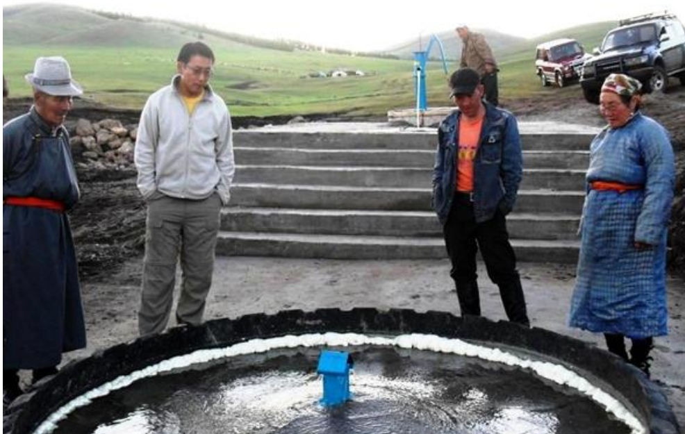
Figure 8. The Ereen project provided domestic and livestock water not previously available in the area.
