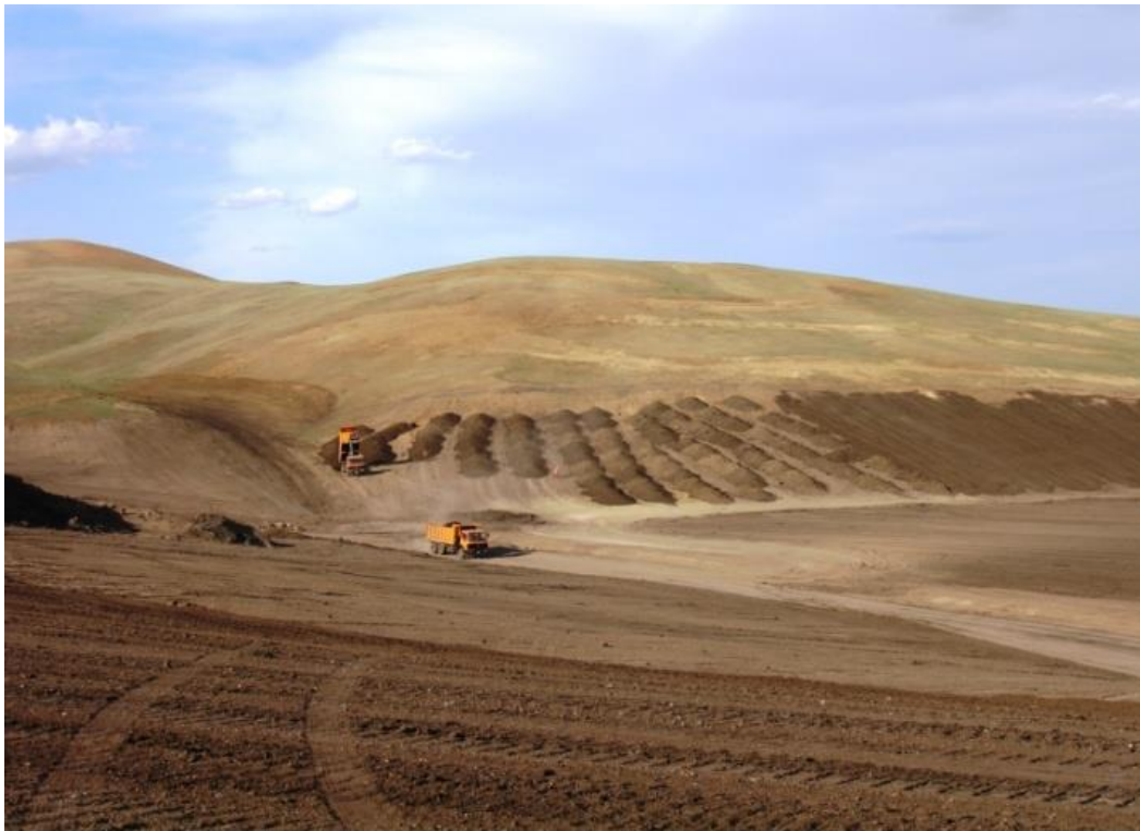
Figure 5. Application of scarce topsoil was completed through an innovative approach.
