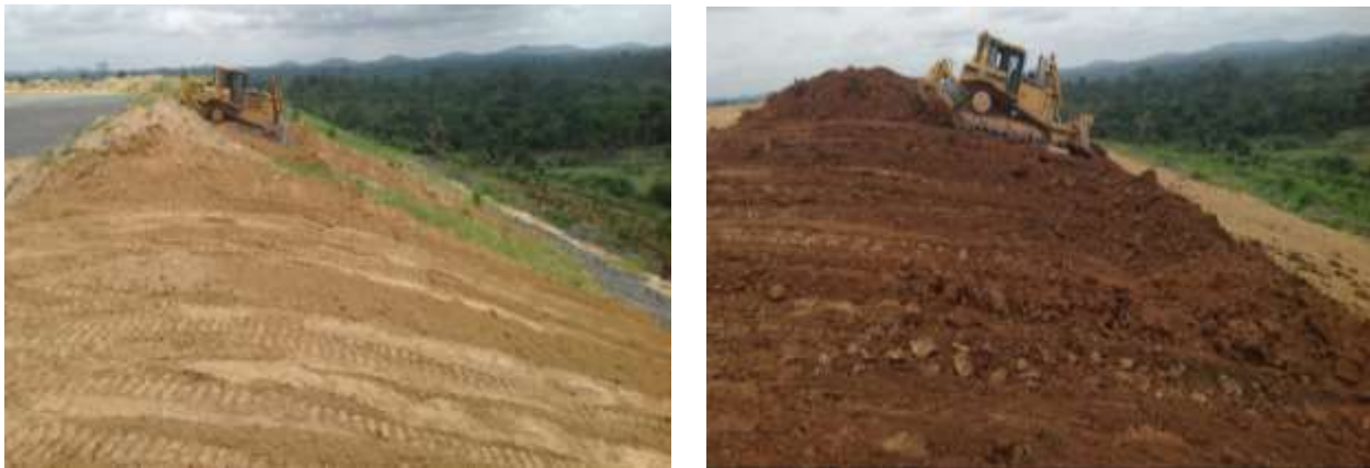
Figure 2. Replacement of stockpiled subsoil (left) and stockpiled topsoil (right).
