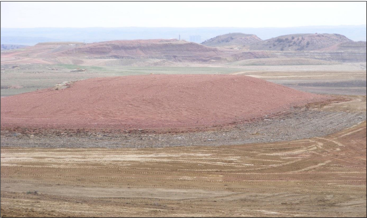
Figure 5. PAR 7A scoria transplant area. Topsoil laydown was ongoing during transplanting.
