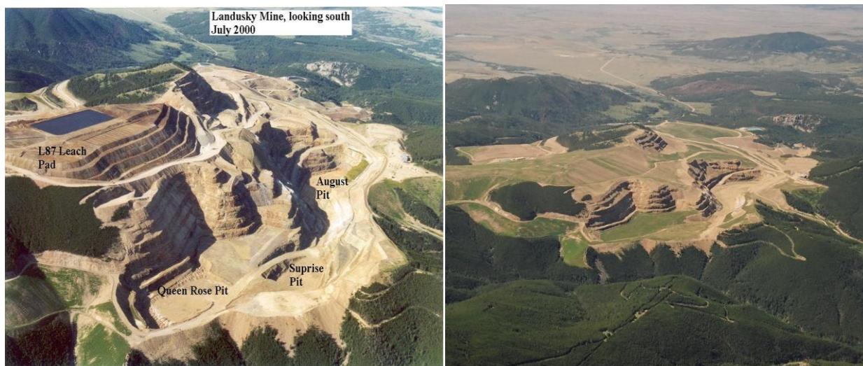
Figure 2. Comparison photos of before and after reclamation of the Landusky Queen Rose-Suprise Pits, 2000-2005. Swift Gulch is immediately below the mine as shown in the picture on the right.
