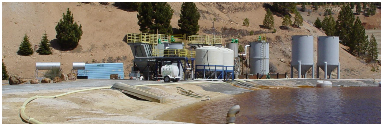
Figure 2. Conventional treatment system at the Leviathan Mine.
