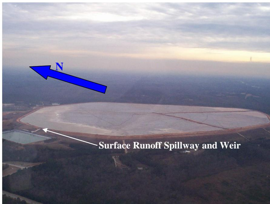
Figure 2. Aerial photograph of the tailings dam (note surface runoff spillway / monitoring location).
