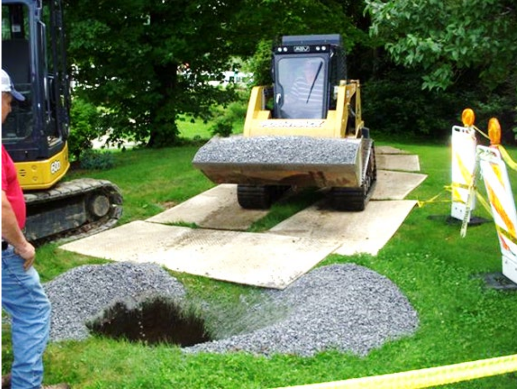
Figure 5. BD Crew in-house project backfilling a pothole subsidence in a residential yard in Allegheny County, Pennsylvania. Total construction cost was $3,112.
