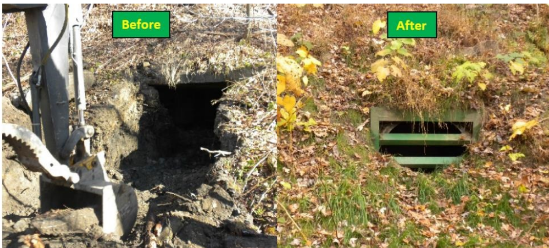
Figure 4. BD Crew in-house project installing a bat gate on an open mine portal in Armstrong County, Pennsylvania. Total construction cost was $2,799.
