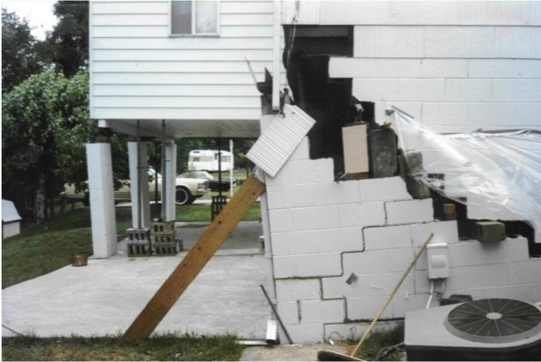
Figure 9. Mine subsidence severely impacting a residence, Allegheny County, Pennsylvania.
