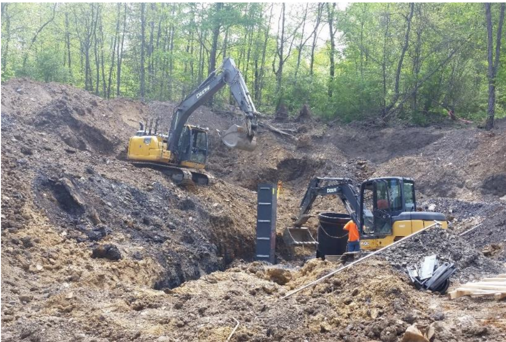
Figure 6. BD Crew in-house project installing a mine drain to prevent mine water from impacting a residential neighborhood in Washington County, Pennsylvania. Total construction cost was $65,000.
