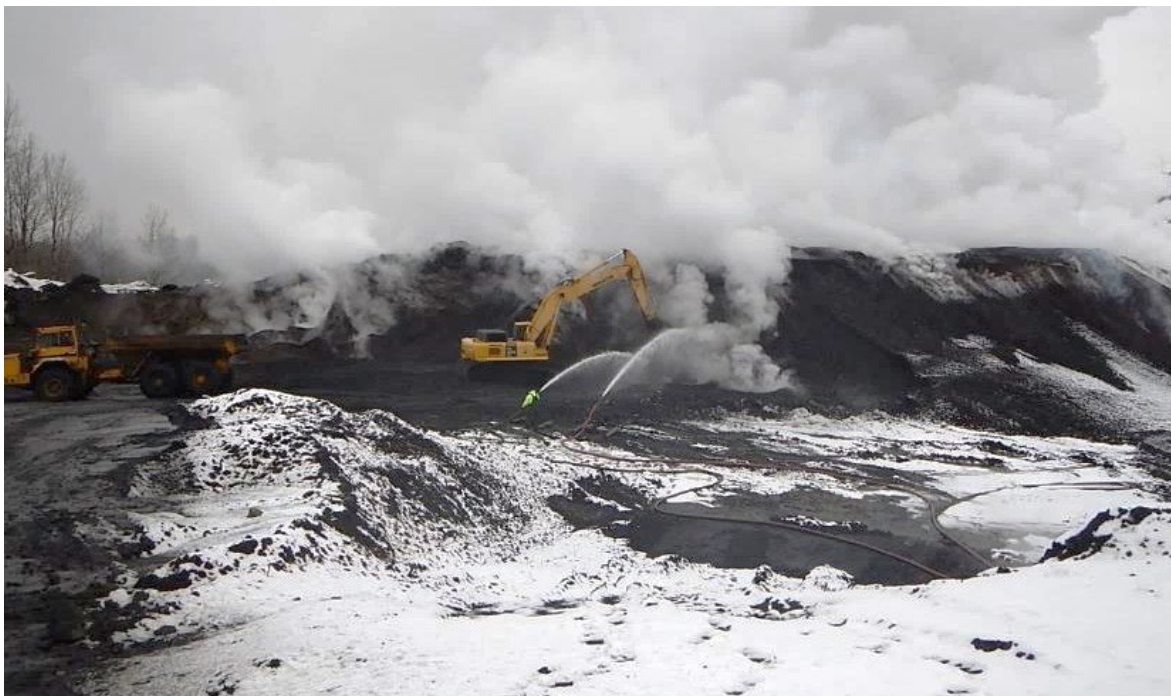
Figure 7. Contracted AML Emergency project to extinguish a coal refuse pile fire in Lackawanna County, Pennsylvania. Total construction cost was $2,213,478.
