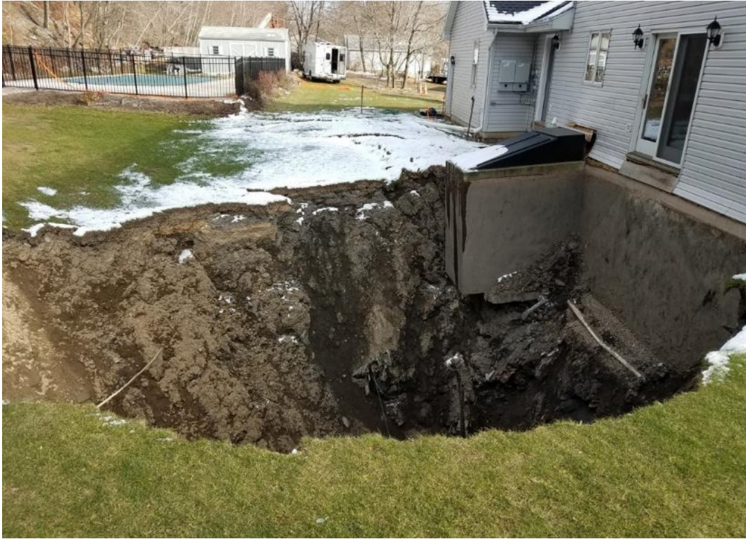
Figure 13. Pothole subsidence threatening a home, Schuylkill County, Pennsylvania
