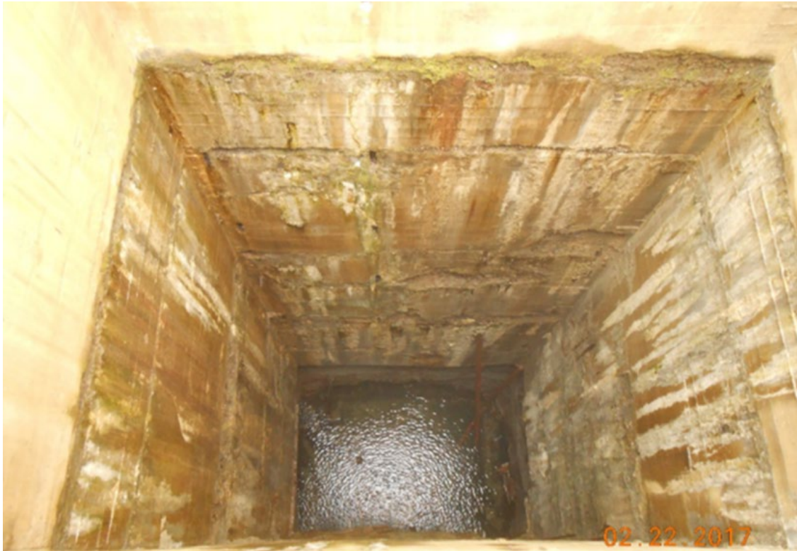
Figure 11. Vertical water-filled mine shaft measuring 12 feet by 16 feet by >60 feet deep, Washington County, Pennsylvania.
