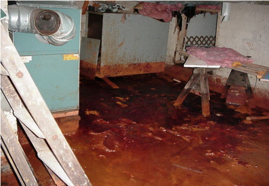
Figure 14. Abandoned mine drainage impacting a residential basement, Fayette County, Pennsylvania.
