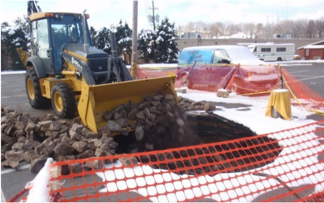
Figure 3. AD Crew in-house project backfilling a pothole subsidence in a parking lot in Luzerne County, Pennsylvania. Total construction cost was $3,190.
