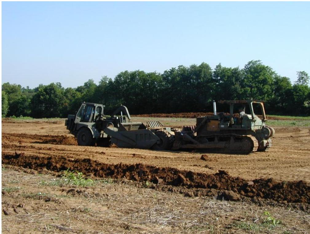
Figure 2. Excavating the experimental soil reconstruction site.
