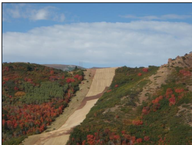
Figure 4 – Blanketed Slope (Colby Reid, 2011)
