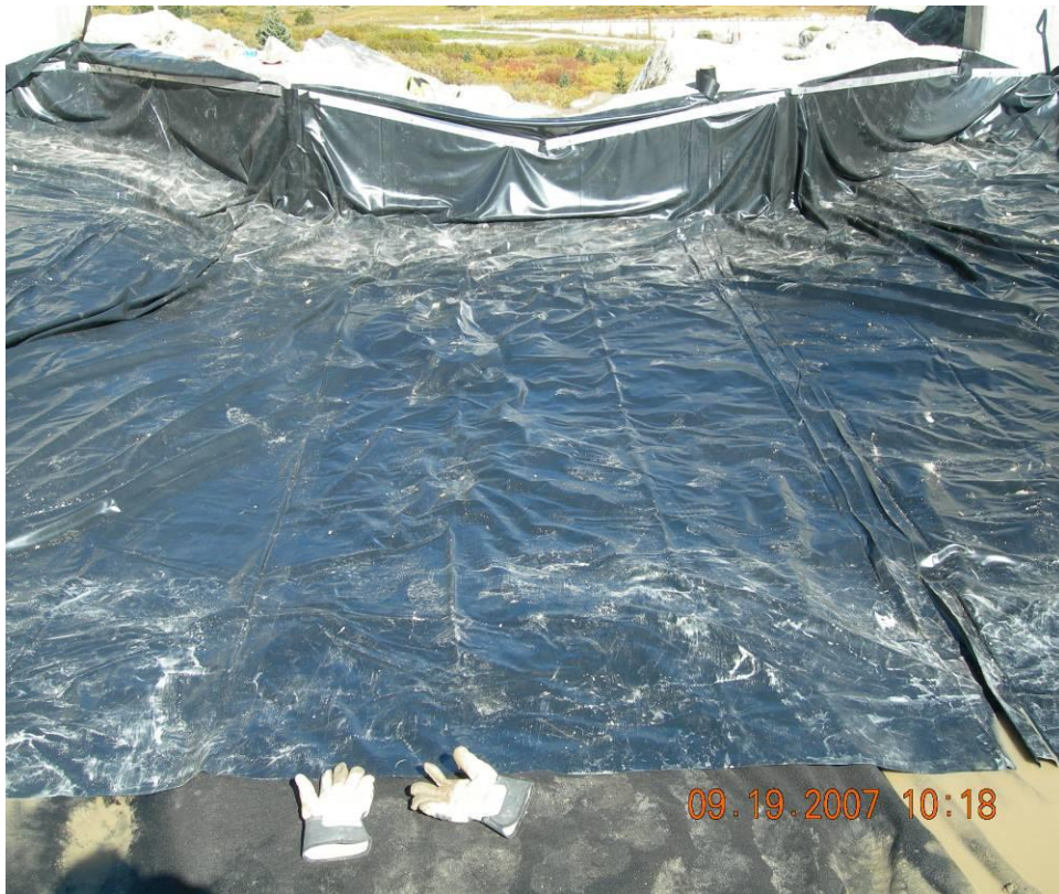
Figure 31. Geomembrane bolted to the retaining wall of the drop structure.
