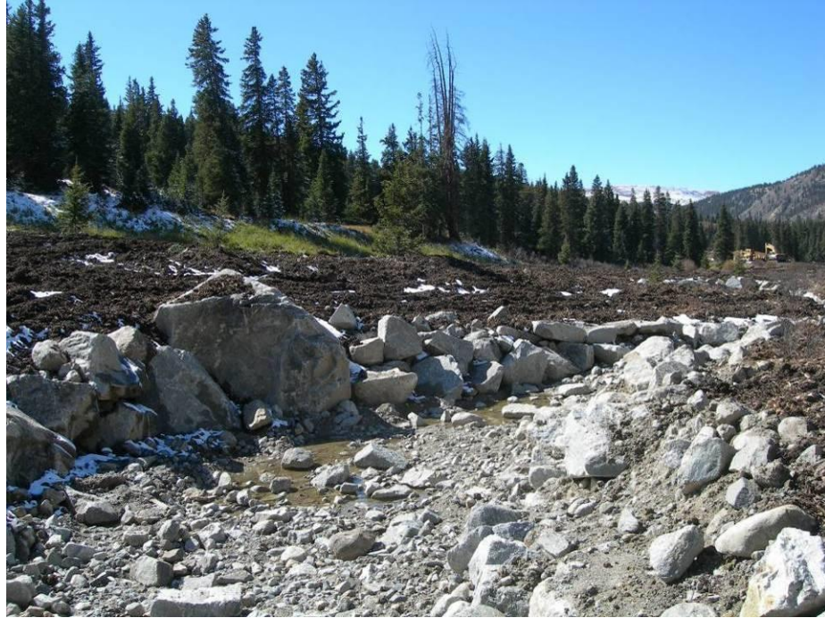
Figure 17. Keystone boulder and armoring at the outside of a meander.
