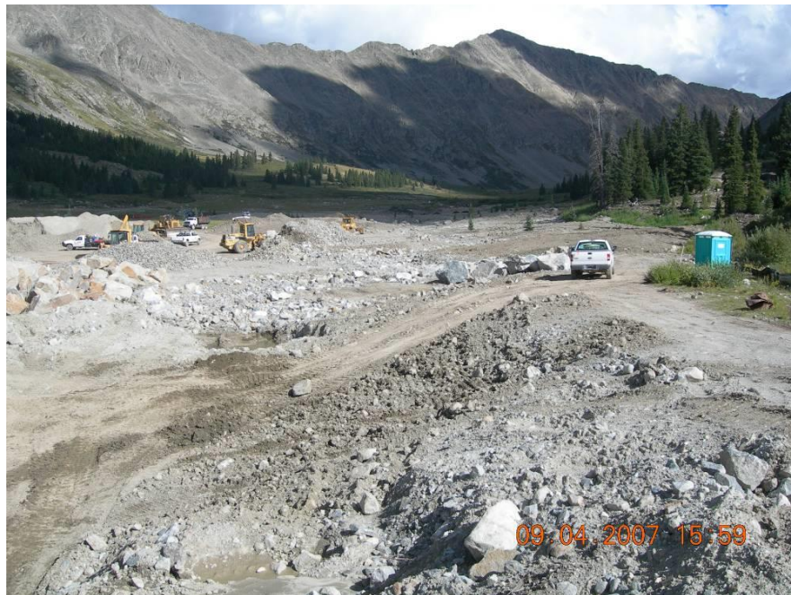
Figure 12. Excavating materials from the downstream channel.
