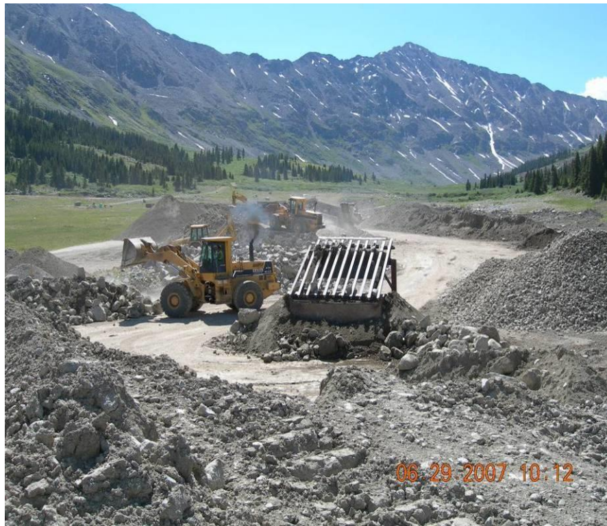
Figure 13. Grizzly operation sorting boulders and finer materials.
