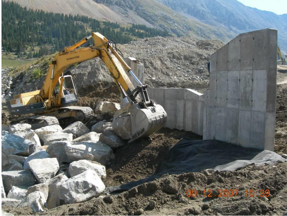
Figure 30. Placement of boulders over bedding materials and geotextile.
