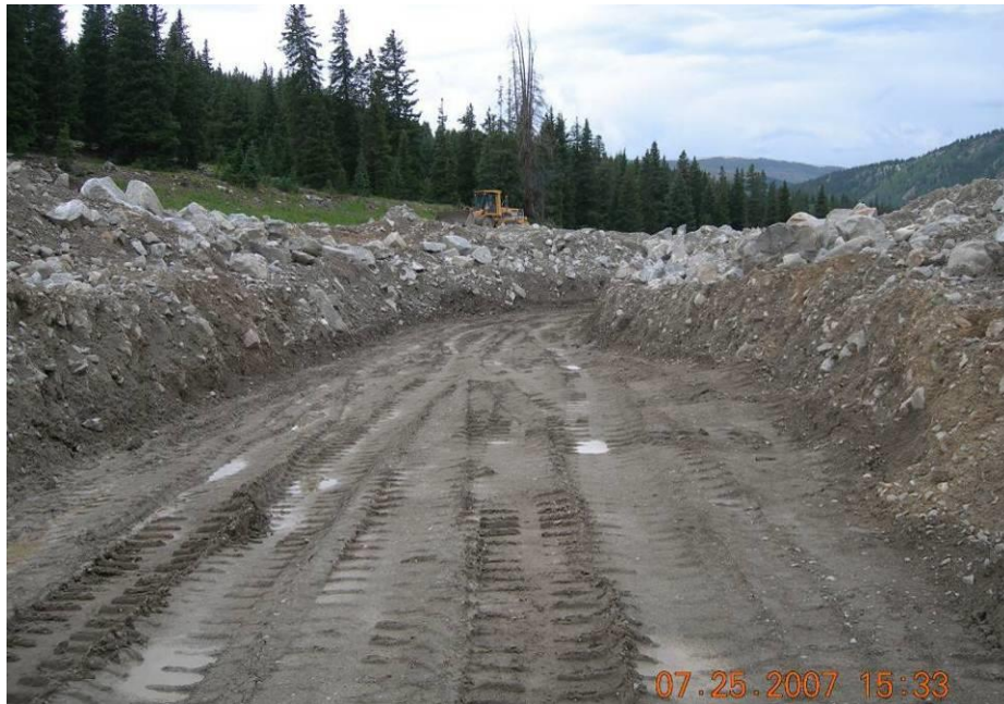
Figure 16. Compacted 2-inch minus material in the Downstream channel.
