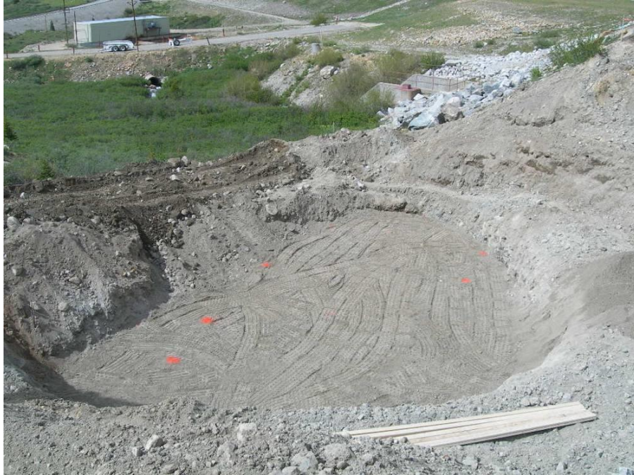
Figure 27. Compacted sub-grade for retaining wall of drop structure.
