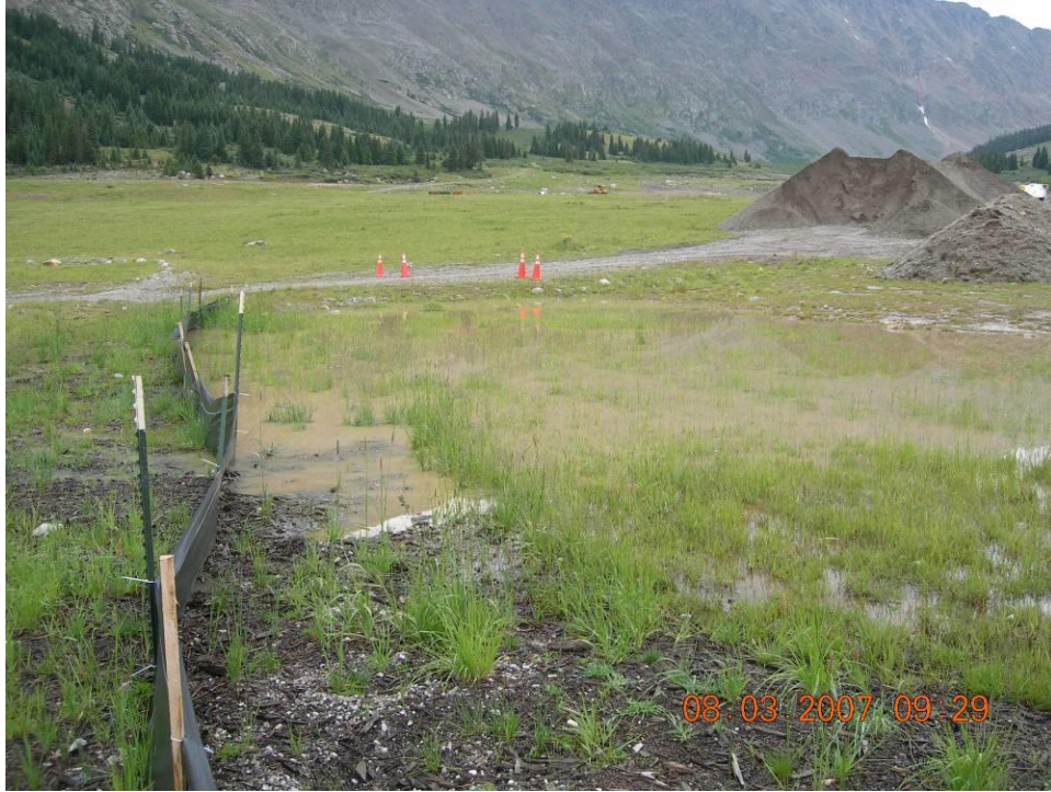
Figure 10. Silt fence along the downstream perimeter of the project site.
