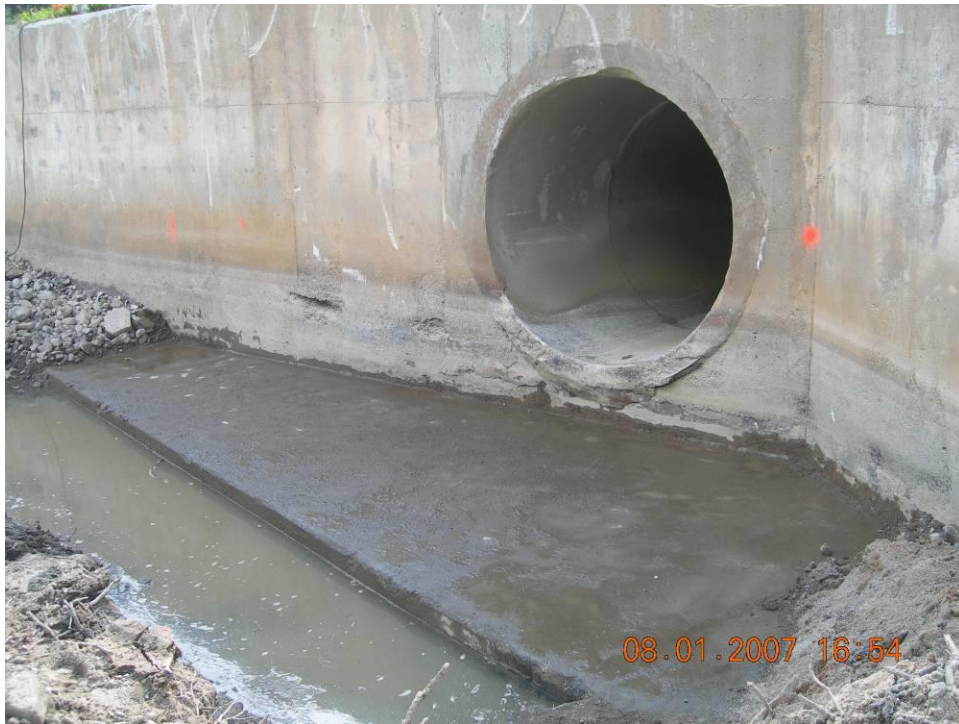
Figure 3. Uncontrolled entrance to the Storke Yard pipeline.
