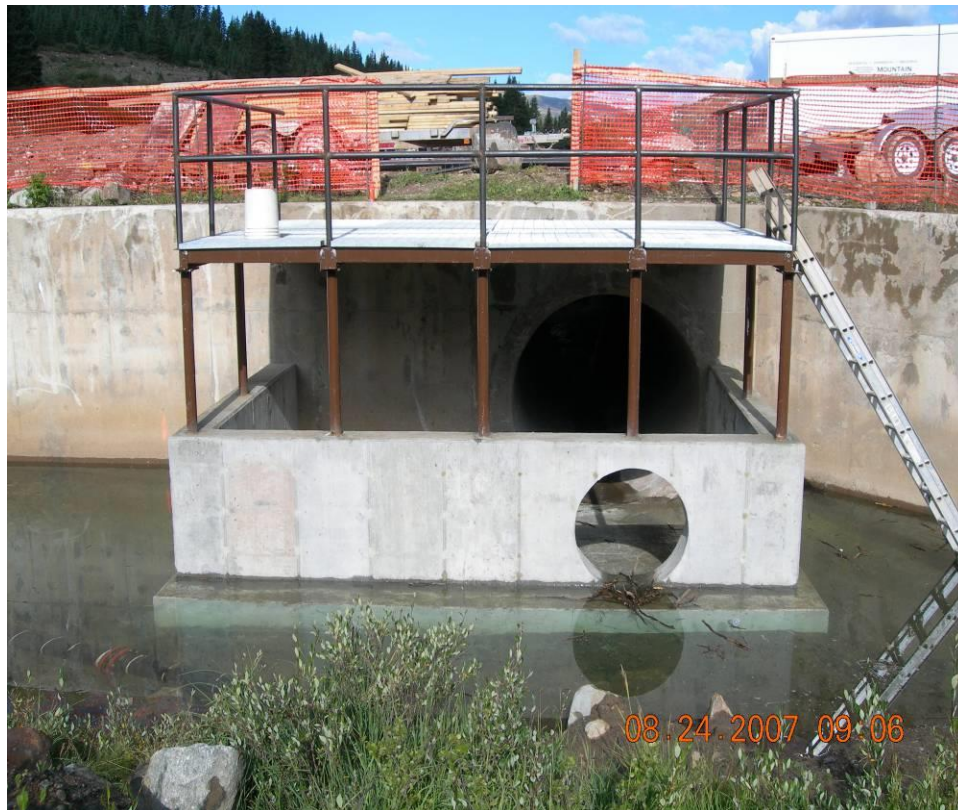
Figure 34. Inlet box with upper steel structure.
