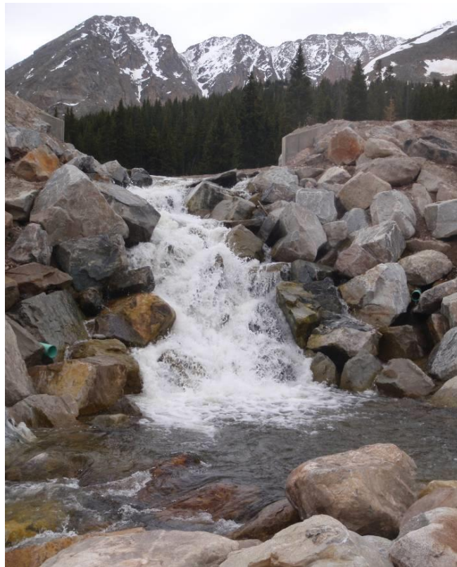
Figure 33. Completed waterfall feature.
