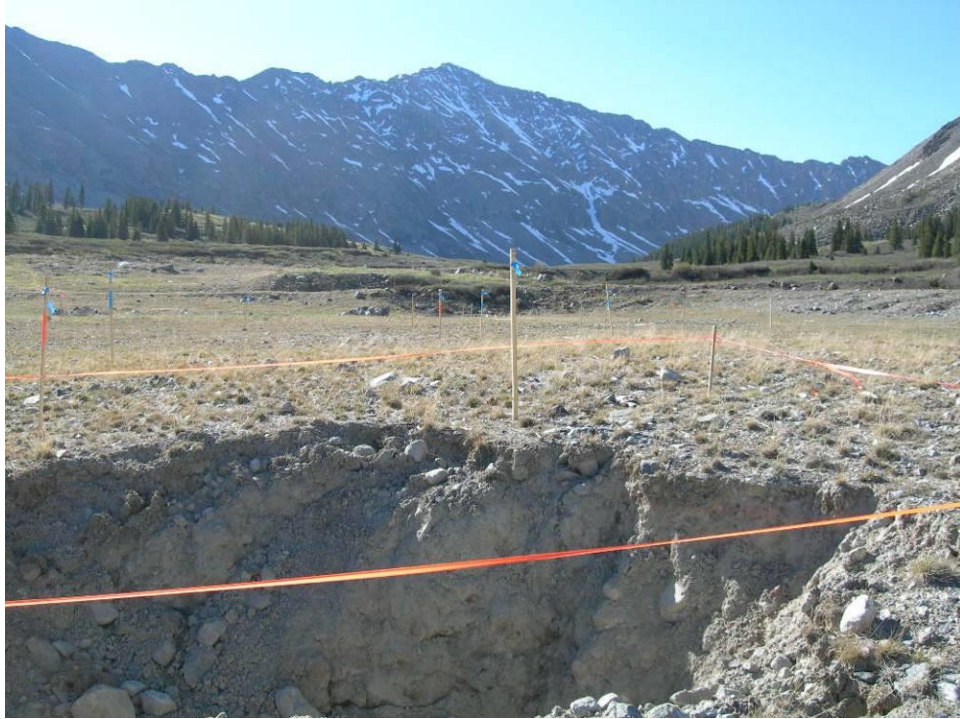
Figure 11. Construction staking in the upstream channel.
