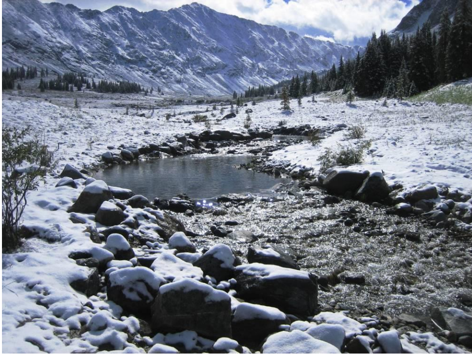
Figure 21. Completed riffle structure.
