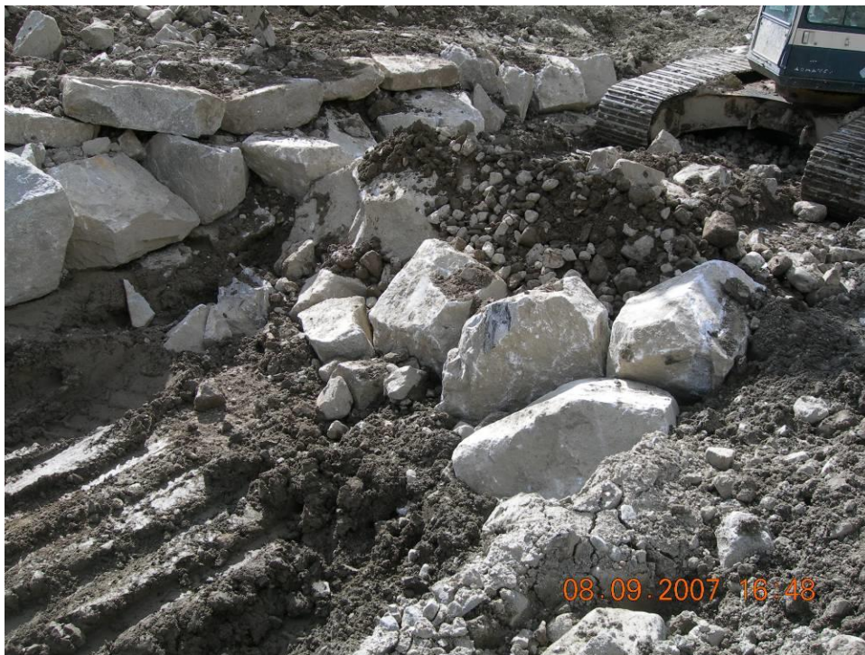
Figure 20. Riffle structure during construction.
