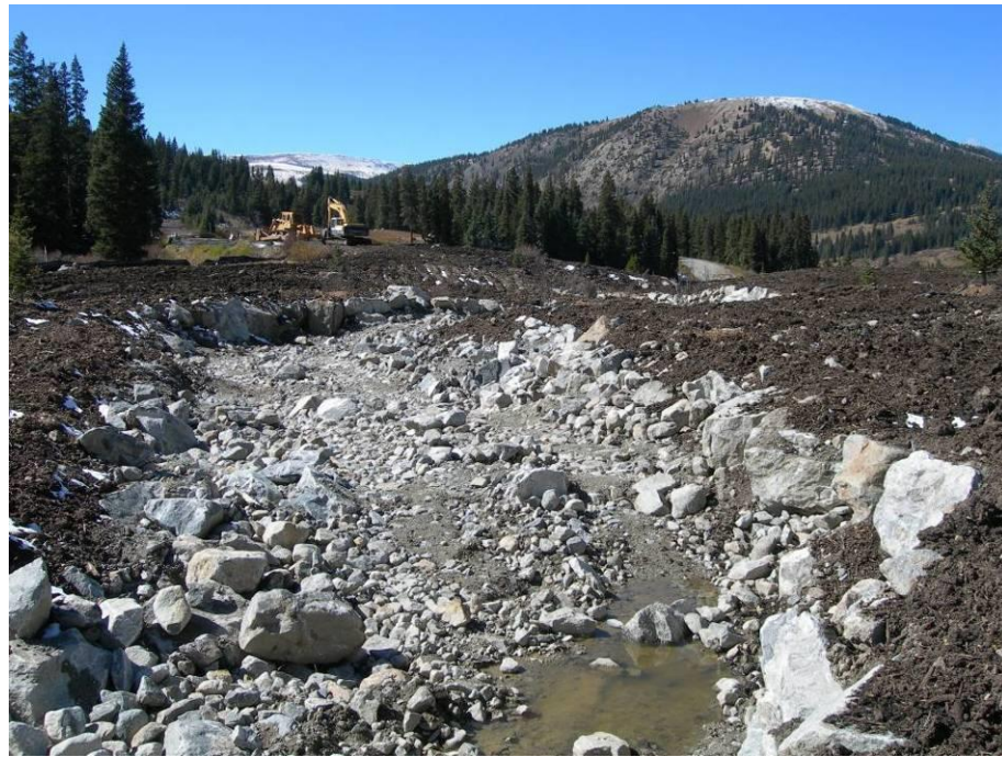
Figure 18. Incised channel will be overtopped by high flows at the inside meander to encourage point bar formation.
