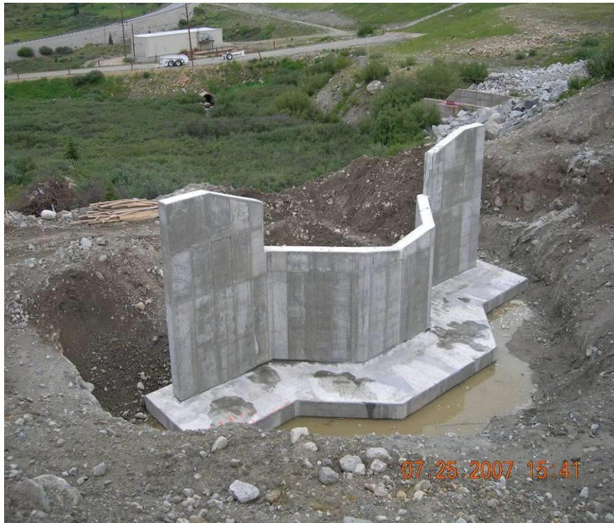
Figure 29. Finished retaining wall during 45-day cure period.
