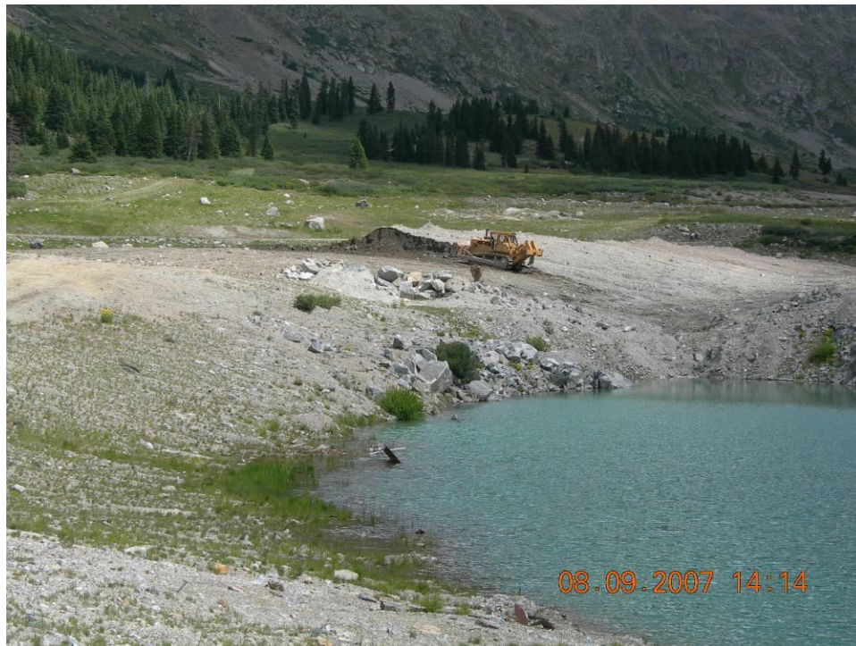
Figure 35. Pushing a materials stockpile into final topography.
