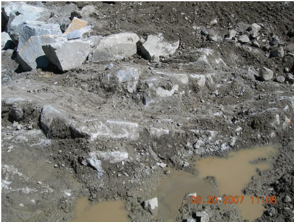
Figure 22. Bedrock outcrop encountered during construction.
