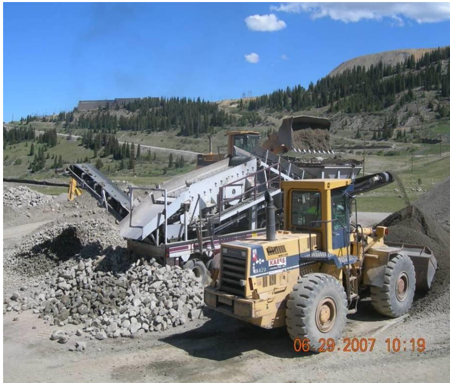
Figure 14. Clemro screening plant sorting 12-inch minus material.
