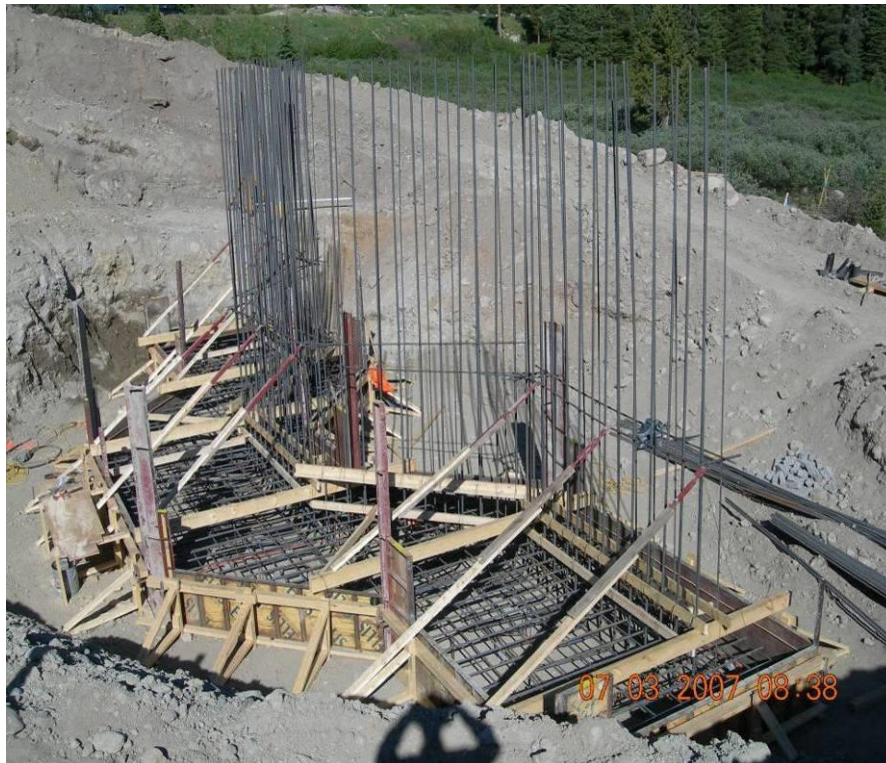
Figure 28. Rebar skeleton of drop structure retaining wall.
