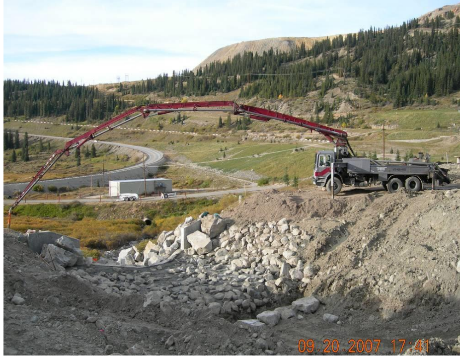
Figure 32. Concrete pump truck grouting drop structure.
