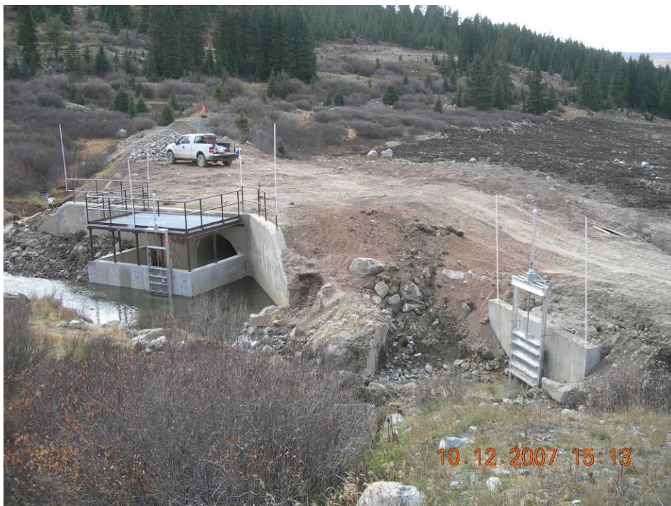
Figure 4. Finished pipe and channel inlet structures.
