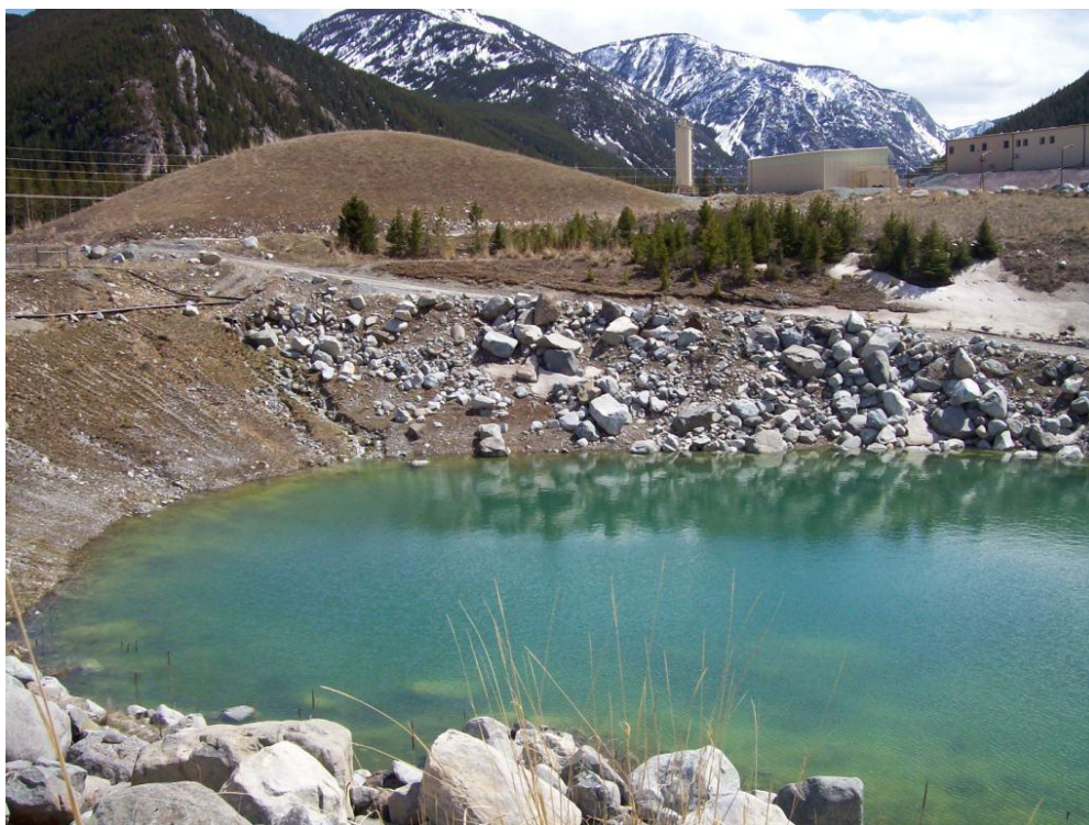
Figure 3. Percolation pond used for disposal of treated mine water. Treated water is discharged to the percolation pond where it infiltrates to the subsurface to ground water and eventually flows to surface water. The percolation ponds at both mines are NPDES-permitted outfalls. DEQ photo.
