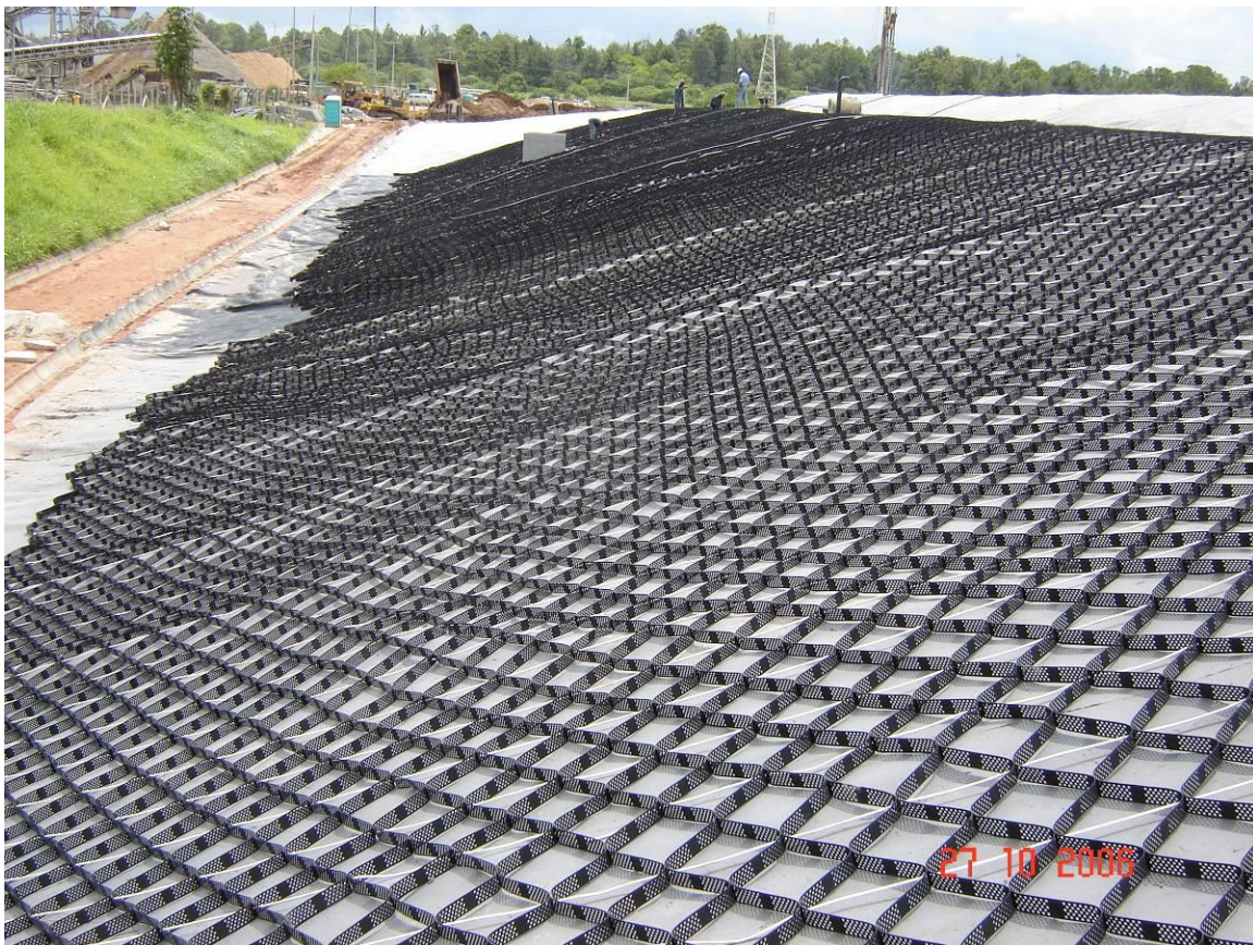
Figure 13. The tendoned geocell system ready for infilling.
