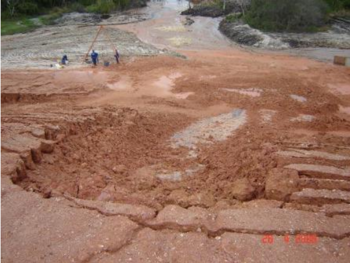
Figure 12. Typical failure of the slope-cover system.
