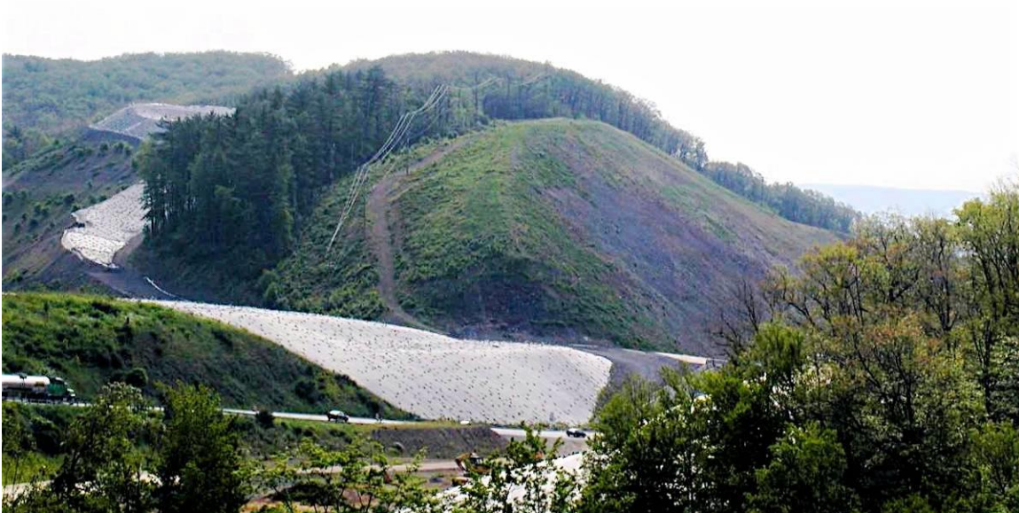
Figure 16. One of many cut faces needing encapsulation.
