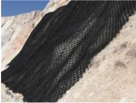
Figure 8. The geocell / geogrid system ready for soil infilling.
