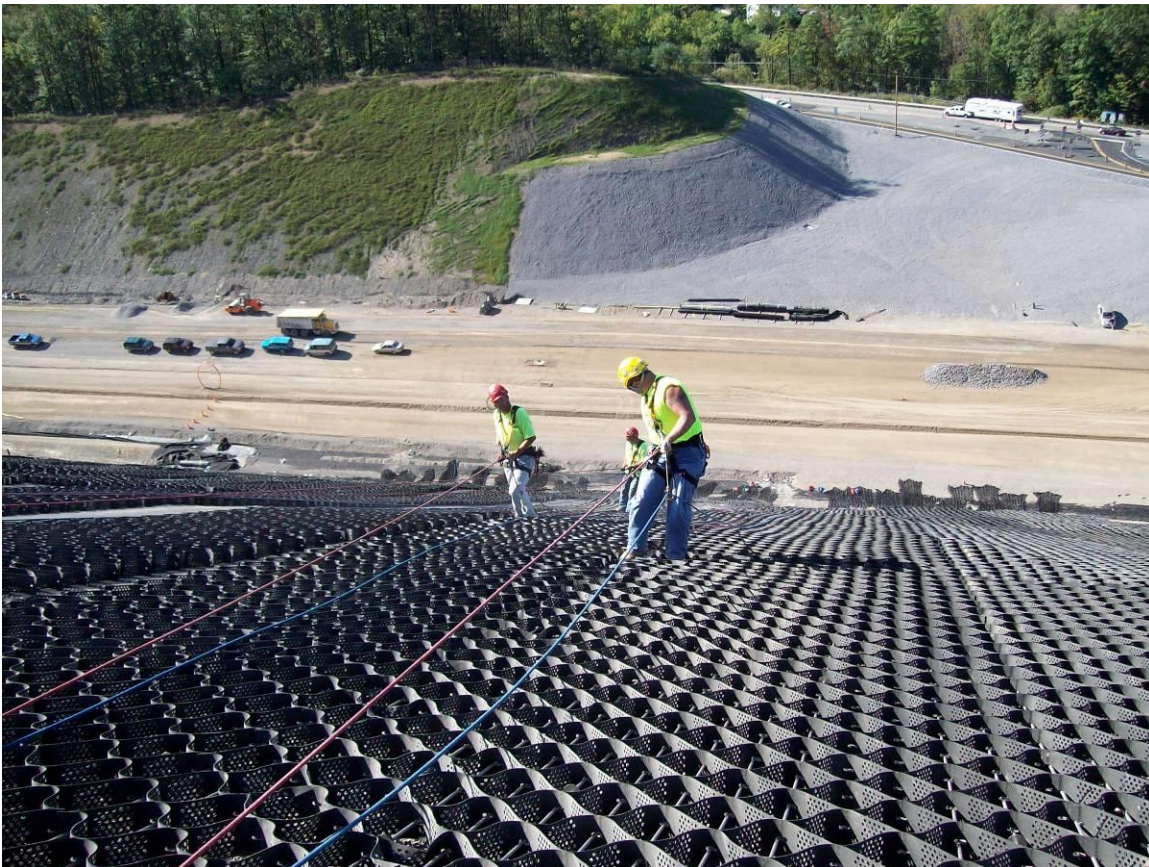
Figure 18. Installation of the geocell on a long steep slope.
