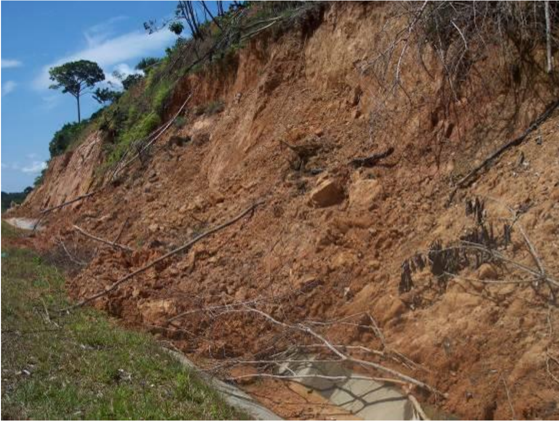
Figure 4. Damages from an unprotected slope along a highway road cut between Iquitos and Nauta, Peru.
