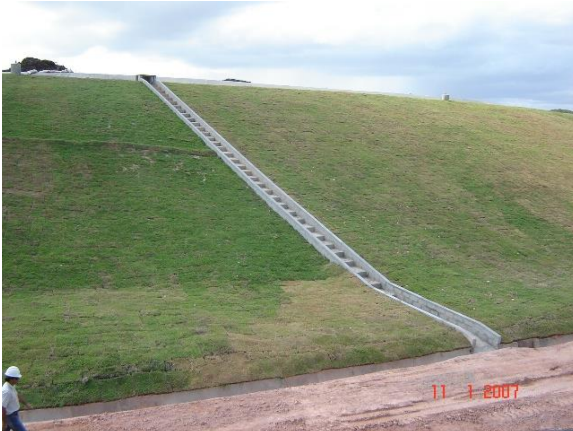
Figure 14. The vegetated system protecting the geomembrane.
