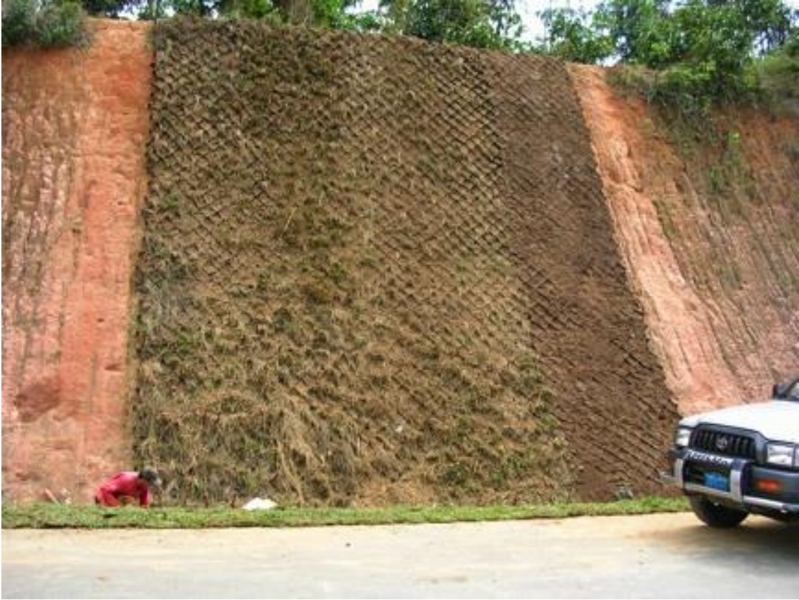
Figure 5. The completed installation of the west slope system on a highway road cut in Peru.
