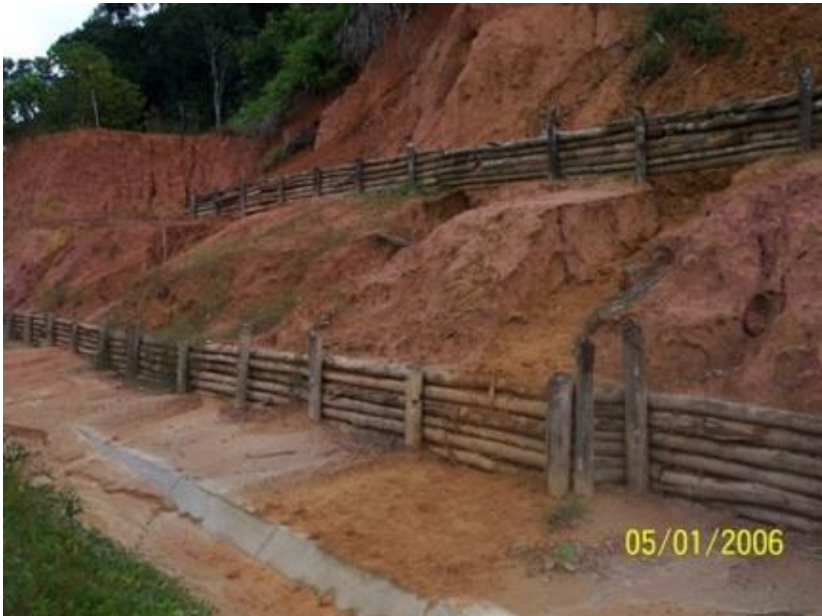
Figure 1. One of many slope surface stabilization schemes which seldom works well.
