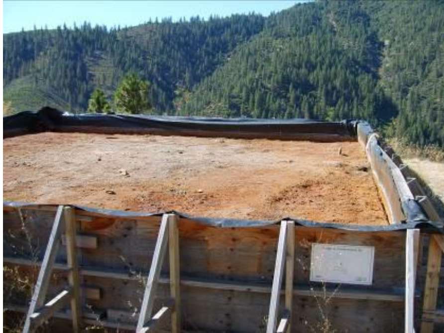
Figure 3. Pilot BCR after being drained and before decommissioning.
