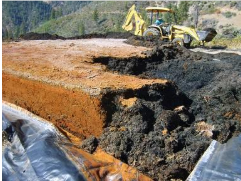
Figure 4. Decommissioning of pilot BCR
