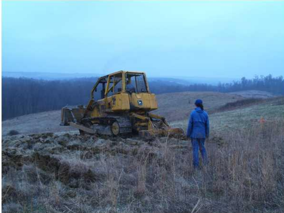
Figure 2. D-6 sized dozer installing ripping treatments.
