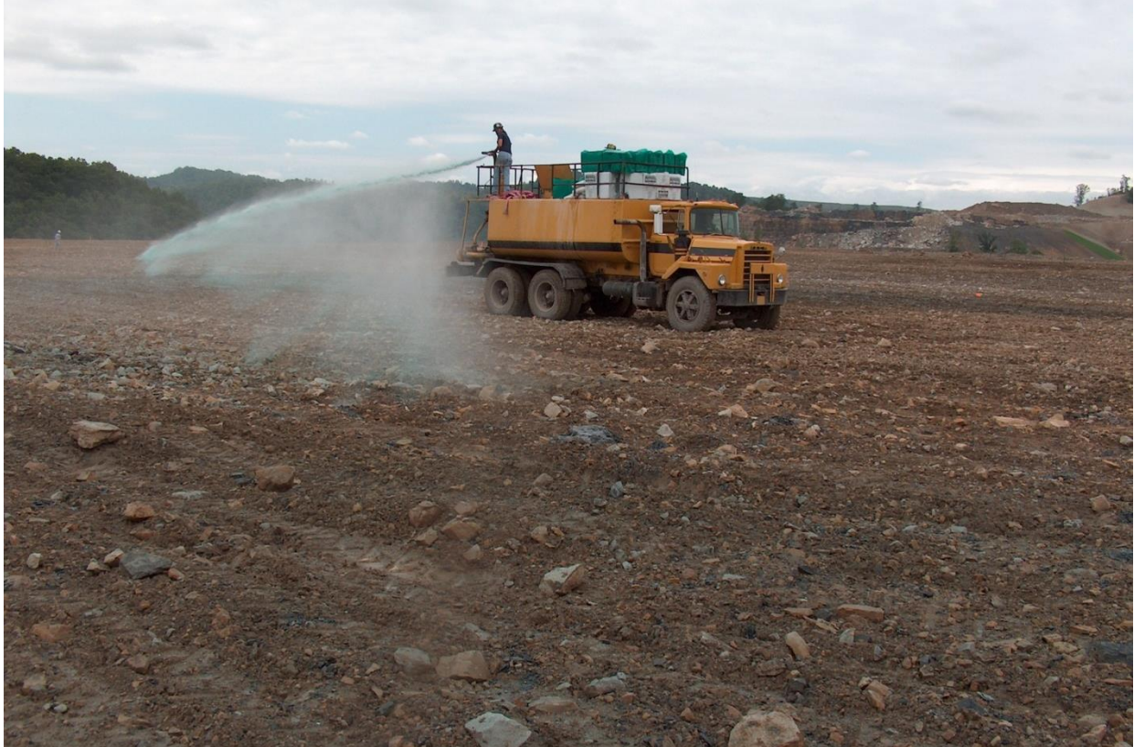
Figure 2: Hydroseeding at Coal-Mac.
