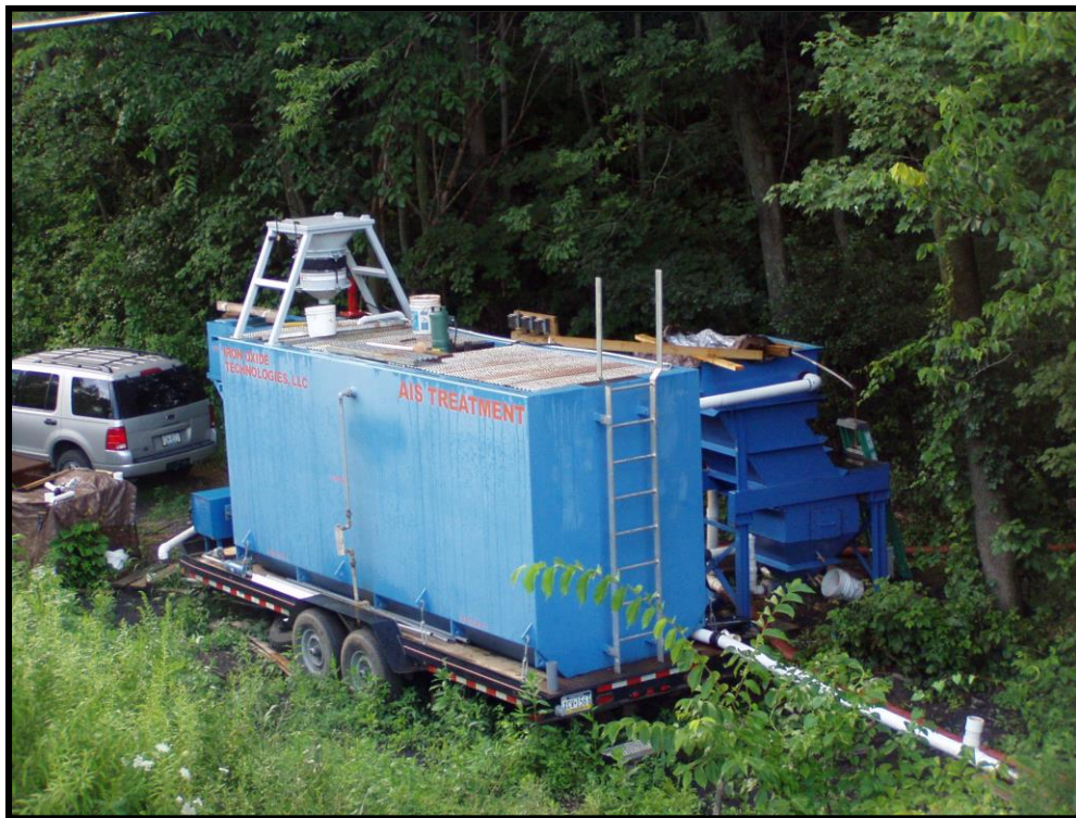
Figure 4. AMD Treatment in a Two-Stage Flow-Through AIS System showing pilot system placed and operating at the Scotts Tunnel AMD Discharge Site.
