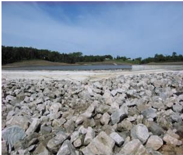
Figure 6. Westercamp II during reclamation
