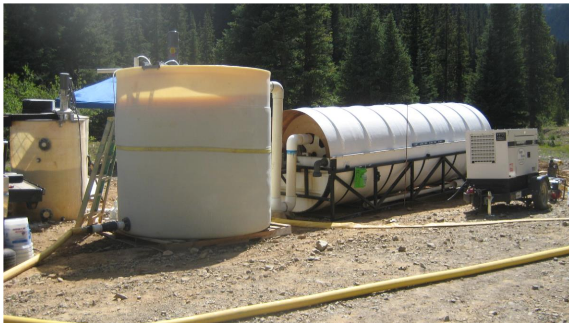
Figure 3: RCTS™ Demonstration System at the Cement Creek Location
