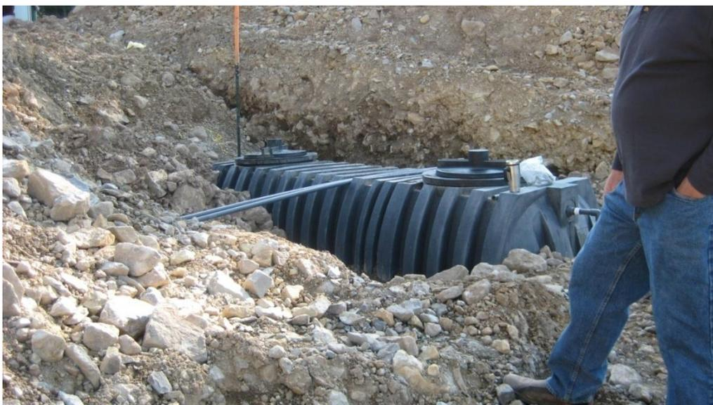
Figure 3. The chitin reactor, housed in a septic tank, prior to burial
