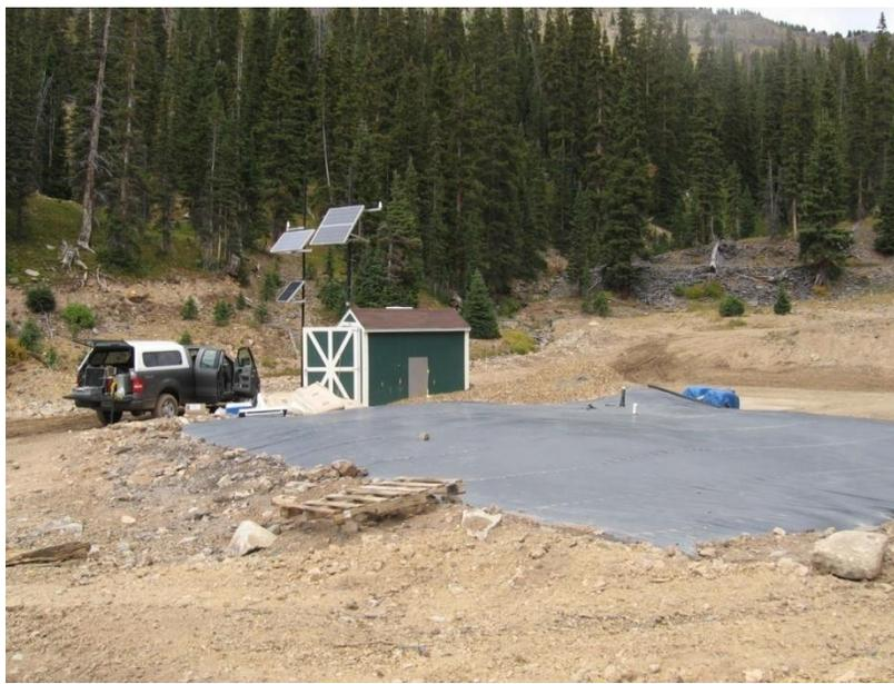
Figure 2. The BCR cell with insulating cover and sampling shed in background
