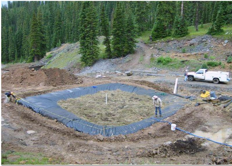
Figure 1. The constructed BCR with exposed substrate
