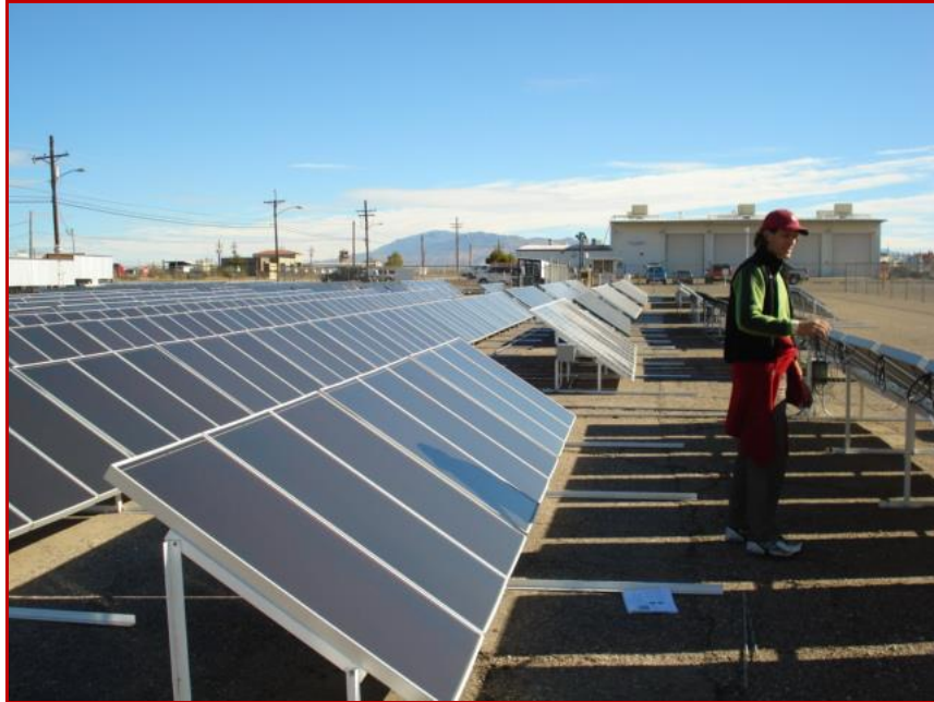
Figure 5: Solar Panel Array – Tucson Electric Power Co. (Unisource, Inc.) test site, Tucson, AZ
