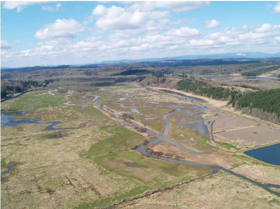
Figure 2. Aerial view showing localized flooding still remained after high flows receded back into the creek.
