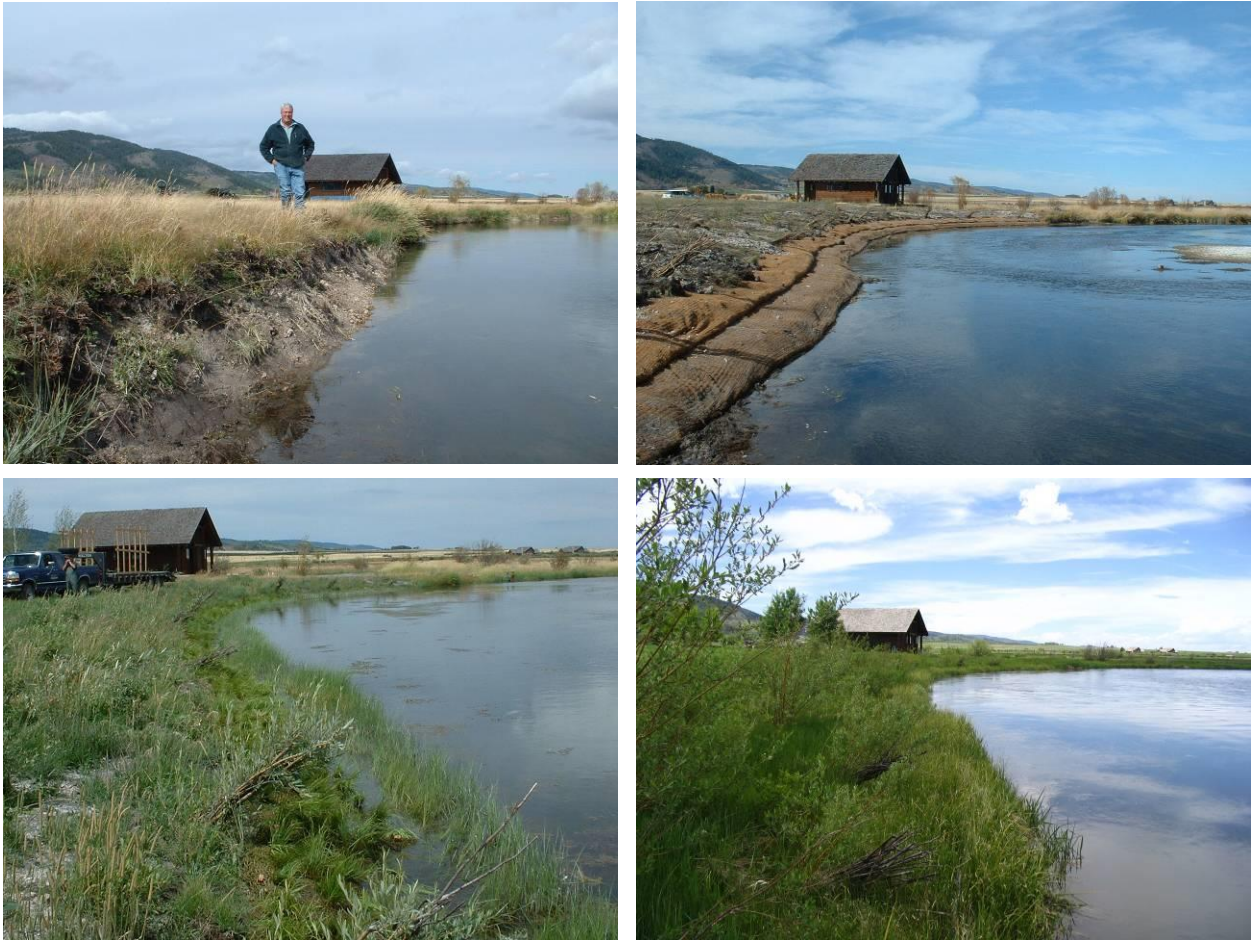
Figure 7. Streambank restoration on the Teton River, Idaho. Top left: Pre-project conditions in October, 2003, featured a steep, eroding bank. The upper bank was dominated by introduced pasture grasses, while the lower bank was barren in most places. In the photograph, a clump of reed canarygrass covers the bank below the building; additional RCG occurs upstream in the background. Top right: The bank was regraded to a gentle slope in October, 2003, and reconstructed with two lifts of soil enclosed in erosion control fabric. Bundles of willow cuttings were planted in the upper bank. Bottom left: Two rows of pre-vegetated coir mats were installed on top of the ECF-wrapped soil lifts and staked into place after high water in July, 2004. This photograph was taken immediately after bank revegetation. In addition to erosion control, the pre-vegetated coir mats provided rapid establishment of native vegetation that could resist re-invasion by reed canarygrass. Bottom right: In July, 2008, native herbaceous vegetation was well established. Occasional RCG plants had started to grow into the lower bank but were very sparse and did not require control. Willows were tall enough to overtop herbaceous potential weeds including RCG.
