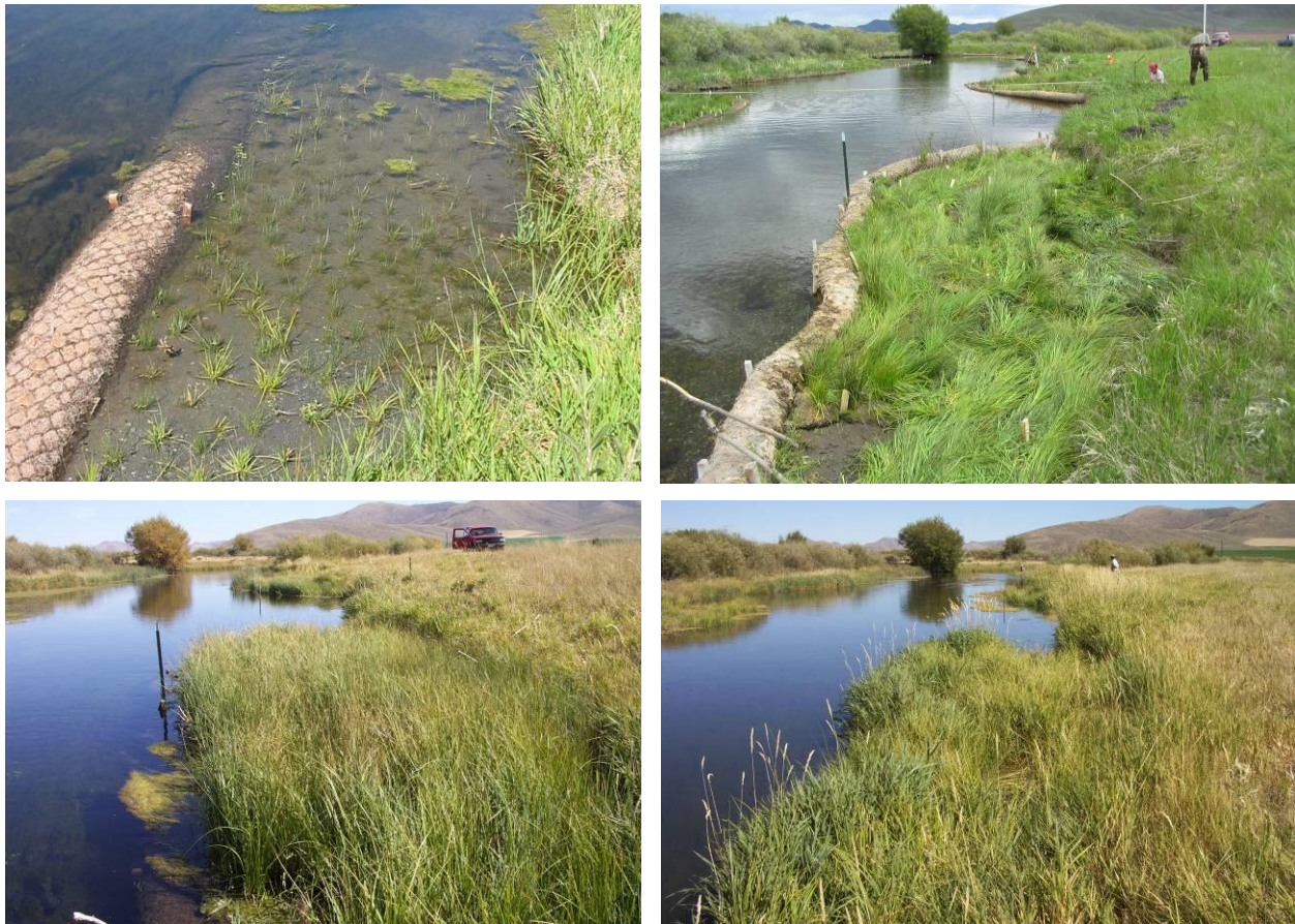
Figure 5. Revegetation of a channel constrictor on Stalker Creek using pre-vegetated coir mats (wetland sod). This site had the highest elevation of the areas revegetated (most fill) and had the most successful establishment of sedge/rush native vegetation and the least muskrat damage. Top left: Unsuccessful establishment of sedge plugs in 2004; mortality increased through spring, 2005. Top right: The same site after installing wetland sod in spring, 2005, at low water. Bottom left: Fall 2005, at high water; nearly full native cover. Bottom right: Fall 2007; native cover remains intact, but reed canarygrass is encroaching from the channel edge after three growing seasons.
