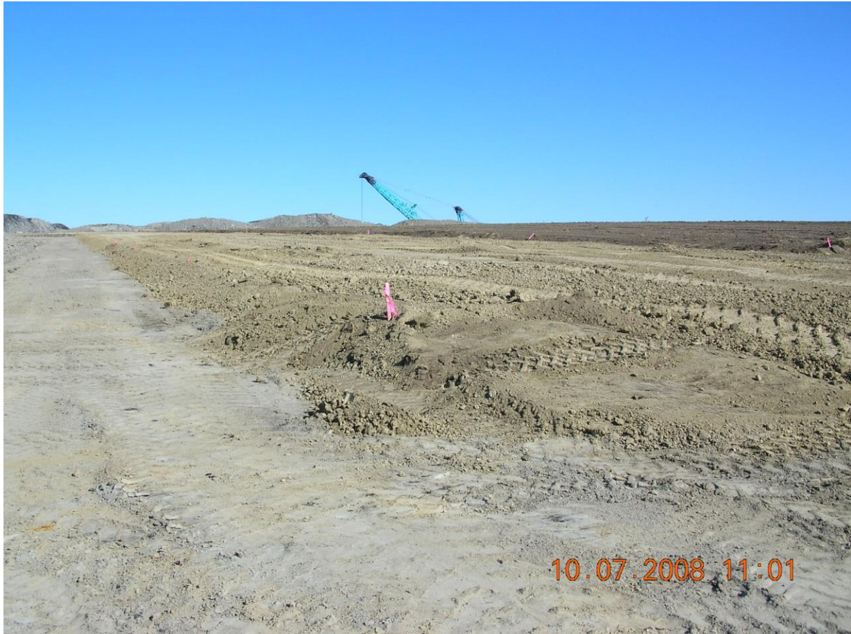
Figure 2. Photograph of subsoil and topsoil redistribution on a grade approval area, looking north-northeast, where subsoil and topsoil has been redistributed progressing from east to west (right to left). Shown on the left on the western edge of the grade approval area is graded spoil; the western edge of the subsoil respread is shown in the center; and shown on the right is the western edge of the topsoil respread.
