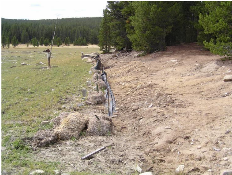
Figure 5. Waste material left in place adjacent to removal area. Run-on from the contaminated area is affecting the reclaimed area.
