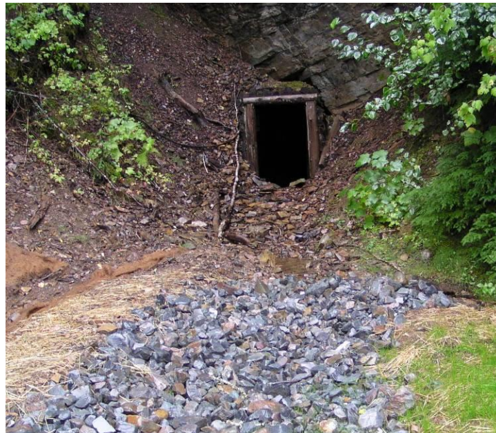
Figure 12. The mine adit closure bulkhead at this reclaimed site is located several feet inside of opening creating an attractive nuisance and risk to site visitors.
