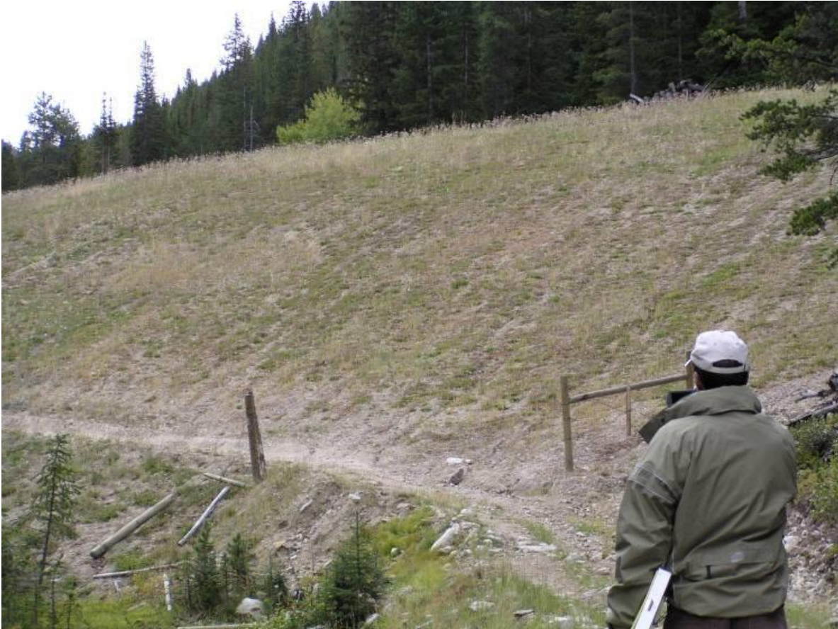
Figure 3. Repository with poor vegetation cover and rills and gullies caused by erosion.
