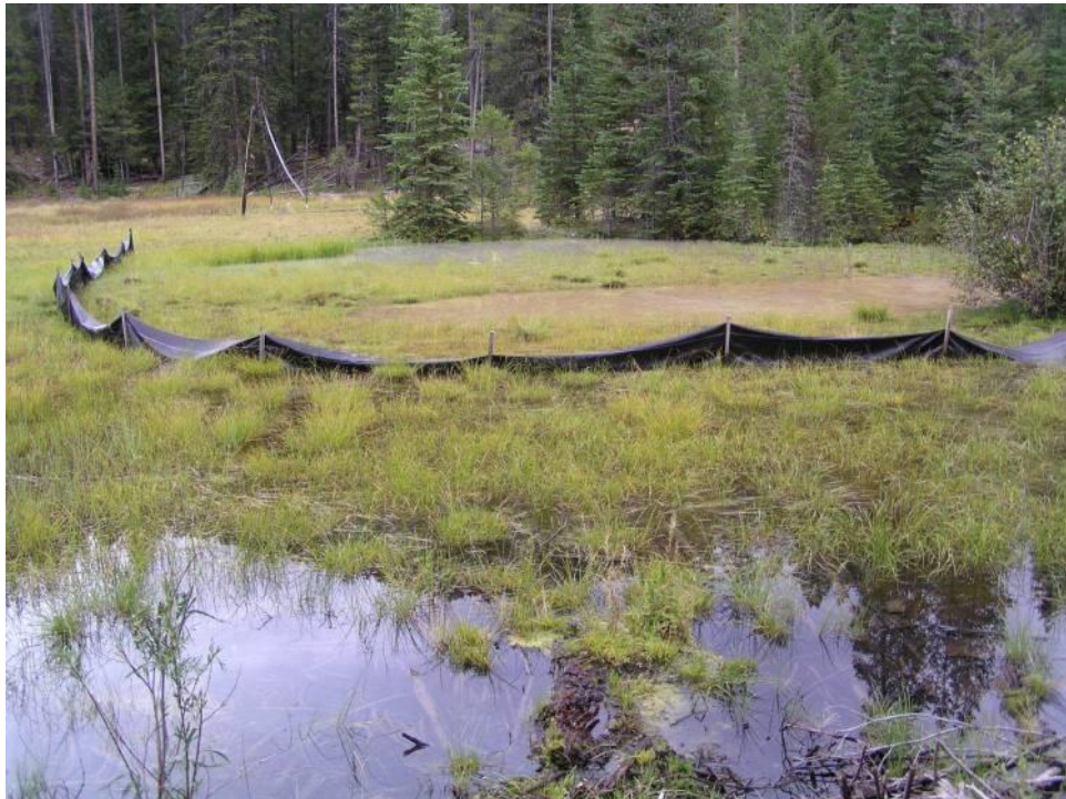
Figure 8. Wetland in a reclaimed area; silt fence needs maintenance or removal depending on erosional characteristics of adjacent area.
