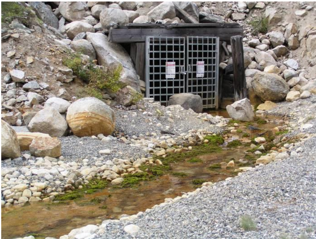
Figure 1. Gated adit protecting public safety, untreated water is a source of acid mine drainage.
