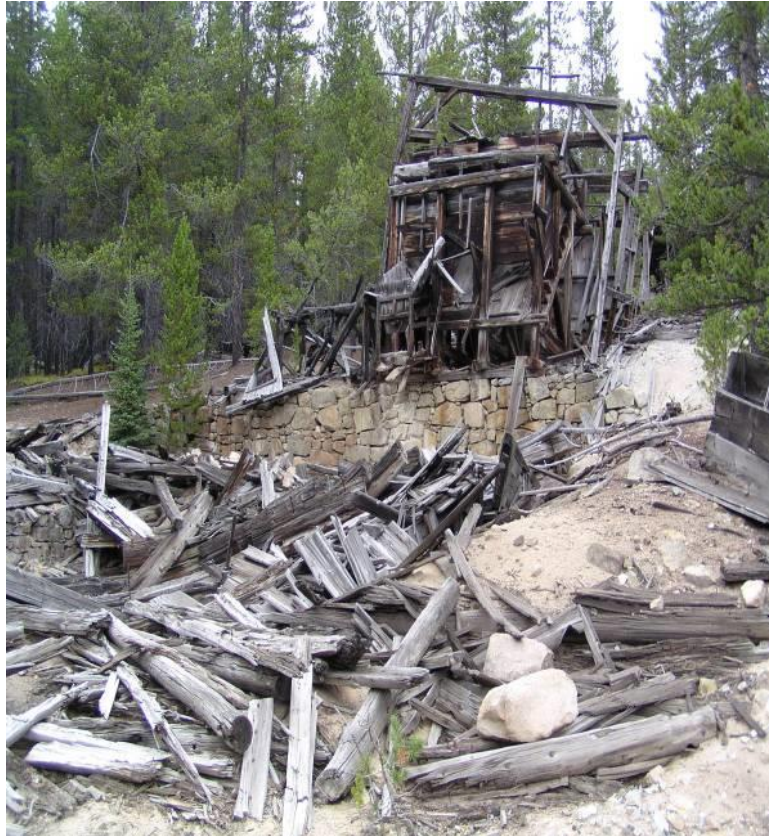
Figure 2. Dilapidated historic structure poses risk to public safety.
