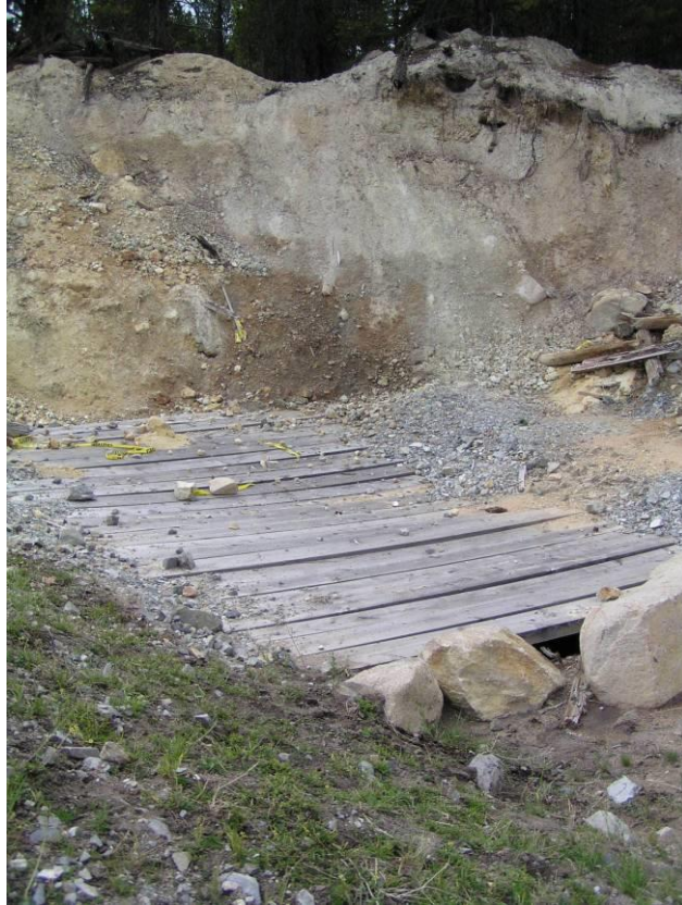
Figure 11. Temporarily closed mine shaft.
