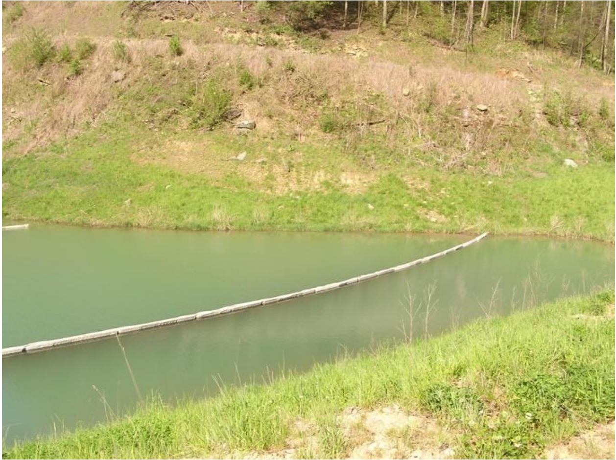
Figure 13. Photo from field inspection verification of pond after treatment.
