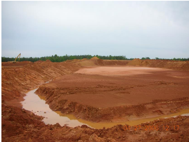
Figure 3: Ring ditch constructed around the inside perimeter of an impoundment.
