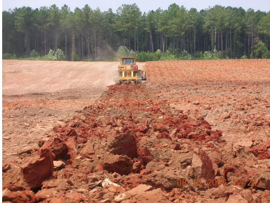
Figure 4: D-8 Deep Ripping
