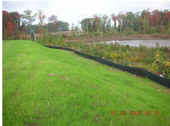
Figure 2: Seeded topsoil and silt fence.
