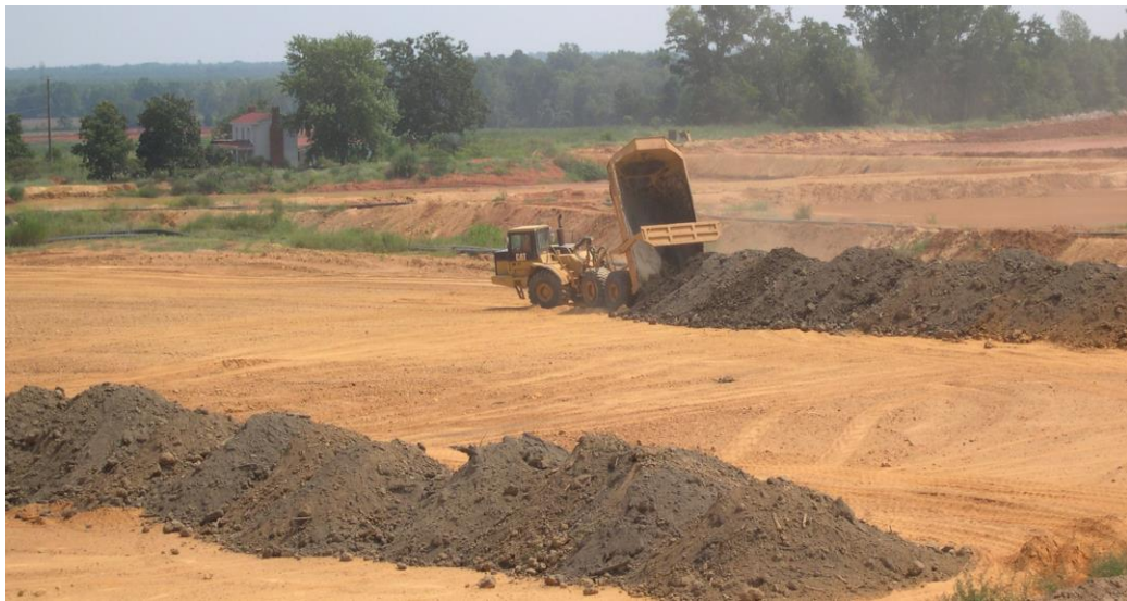
Figure 5: Topsoil returned in windrows
