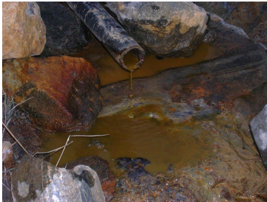
Figure 2. Low flow from the effluent pipeline of the experimental bioreactor at Black Hawk, CO, on November 10, 2007. Effluent flow was originally ~36-lpm.
