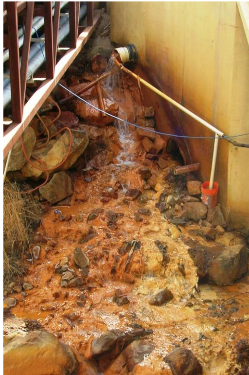
Figure 1. MIW discharge from the National Tunnel adit into Clear Creek at Black Hawk, CO.
