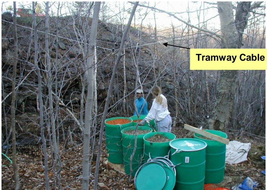
Figure 4: South Cut BCR system construction. A tramway cable arrangement was used to transport materials from a staging area to the treatment site.
