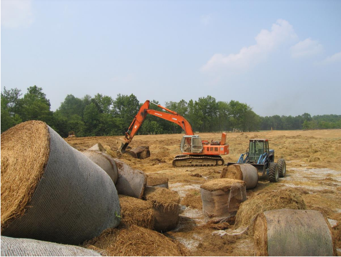
Figure 6 – Placement of the Compost Layer: Enos loop Wetland - West VFP.
