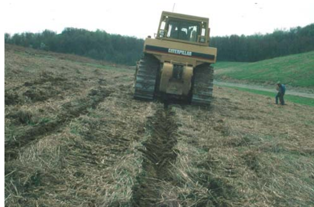
Figure 2. Ripping treatment along the contour.
