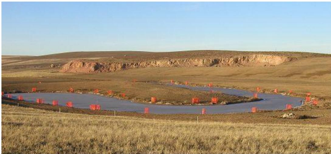
Figure 8: Avocet Reservoir on Reclaimed Tisdale Creek at Caballo Mine with Reconstructed Scoria Bluff and Trees with Protective Fencing (S. Storie, 2003).
