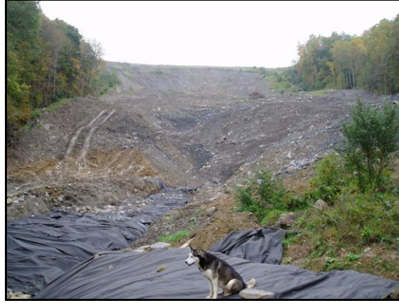
Figure 17: Particle Size Distribution at the Toe of Fill 1. The photograph was taken by KYDEP during new underdrain installation in October 2006.
