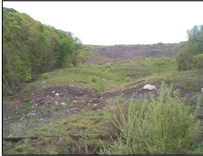
Figure 15: General View of Landslide on Durable Rock Fill, Looking Upslope from Toe. (Photograph taken in April 2005).
