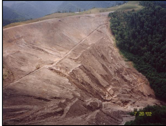
Figure 12: Erosion and Sloughing on Fill Face from Uncontrolled Storm Runoff.
