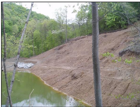
Figure 19: Close-up of Colluvium and Weathered Bedrock Near Toe of Fill 1. (Photo taken in April 2005).
