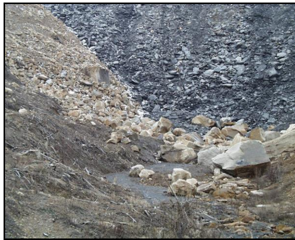
Figure 11: Comparative Effectiveness of Gravity Segregation between Sandstone and Shale Particles at Toe of Durable Rock Fill Under Construction. (Photo taken in spring 2000 during the EIS stability study).
