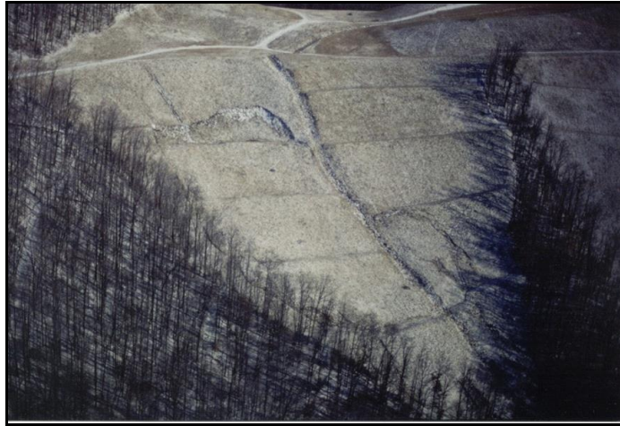
Figure 10: Translational Land Slips on a Durable Rock Fill. (Aerial photo taken in December 1999 during the EIS fill stability study).
