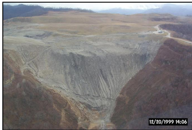
Figure 14: Durable Rock Fill Lacking Contemporaneous Reclamation.
