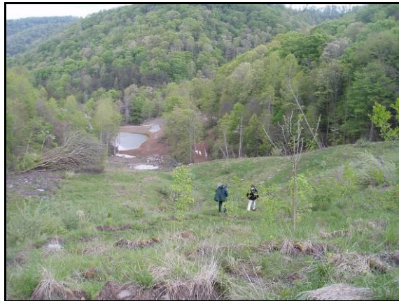
Figure 18: View of Toe and Settlement Pond from the Outslope of Fill 1. Exposure of thick colluvium and weathered bedrock occurs to the right of the pond. (Photo taken in April 2005).
