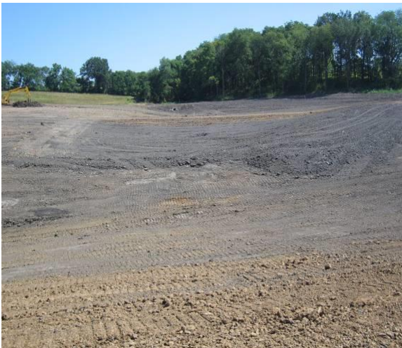
Figure 7. Pond being reconstructed.
