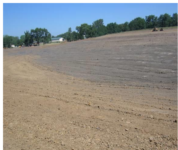
Figure 8. Pond and terraces being reconstructed.
