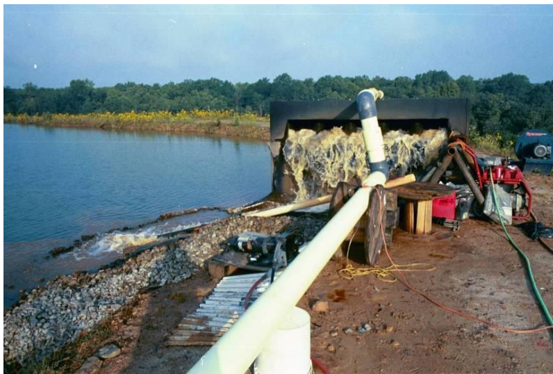
Figure 9. The 7.56 million L (2 million gallons) per day Maelstrom Oxidizer
