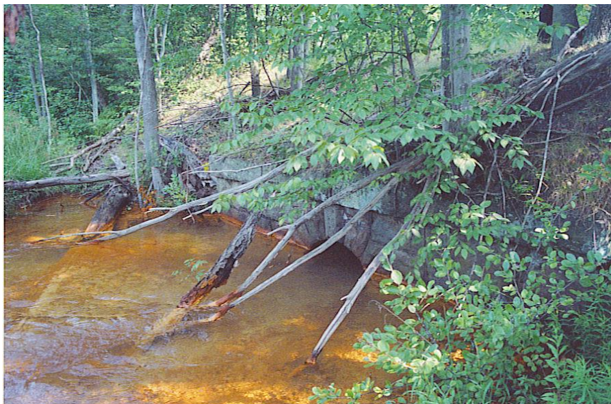
Figure 4. Dundee Outfall---Nanticoke Creek
