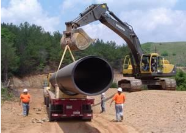
Figures 3B and 3C. Installation of 63” Diameter HDPE Pipe to Divert Belltown Creek.
