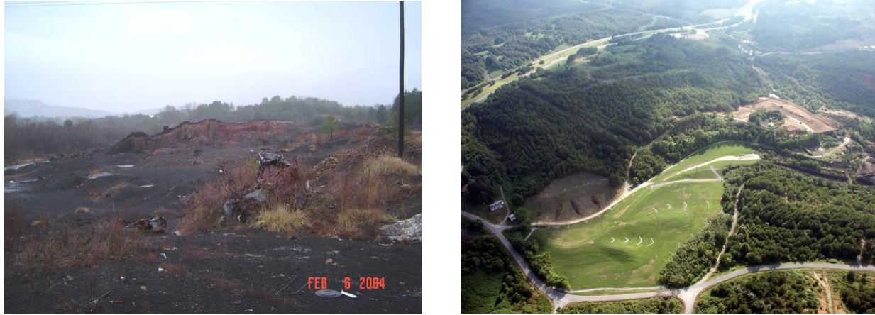
Figure 9A and 9B. Before and after Photographs of the Ellis Branch Slag Cap
