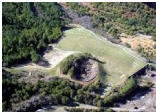
Figure 6B. Completed Containment Cap
