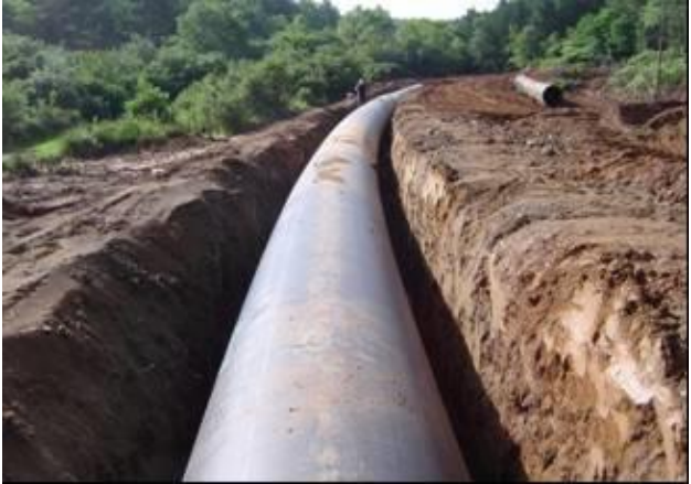
Figures 3B and 3C. Installation of 63” Diameter HDPE Pipe to Divert Belltown Creek.
