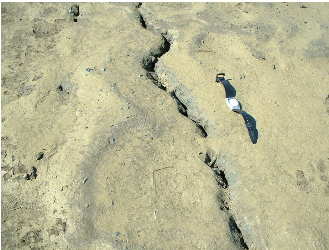
Figure 7. Cracks on the Co-Mix cover of Cell #5.
