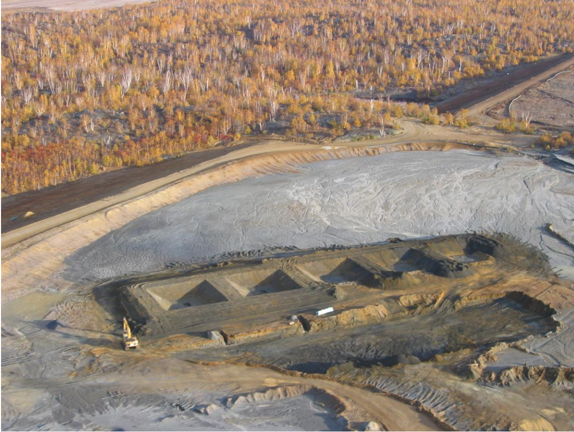
Figure 4. Aerial view of the first phase of construction.
