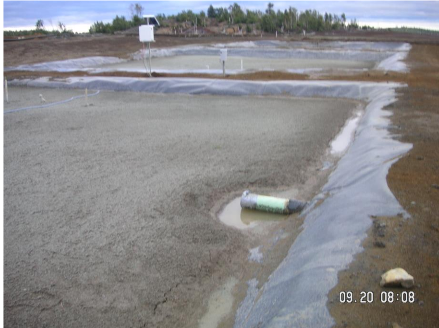
Figure 6. Lysimeter L3 with the topsoil cover.
