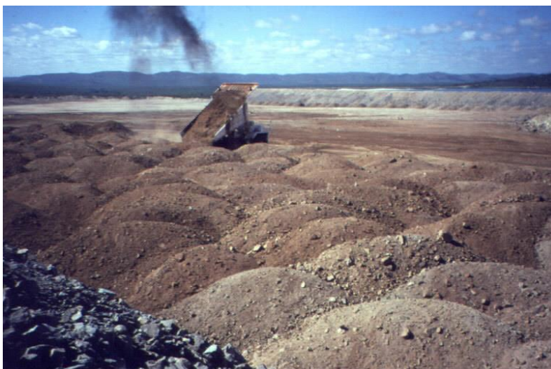
Figure 2. Placement of rocky soil mulch layer on South Waste Rock Pile cover trial.
