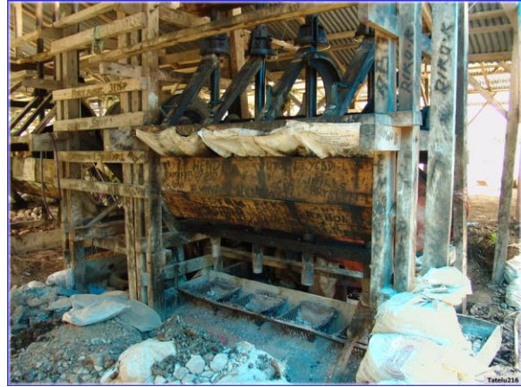
Figure 9. Atop each rod, or stamp, is an eccentric wheel that raises then drops the stamp to crush the ore in bins beneath.
