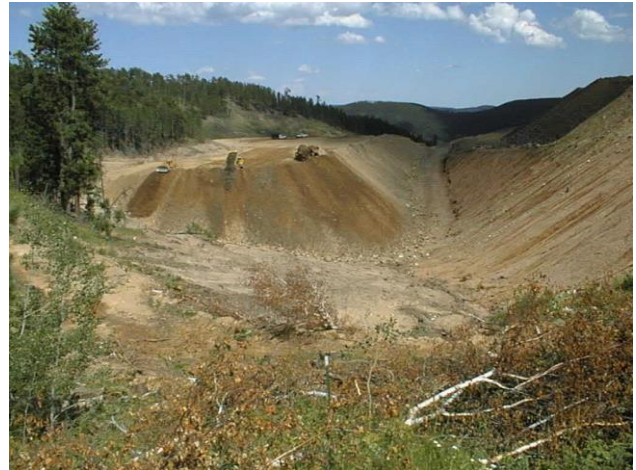
Figure 4. Hauling rock into N-valley tributary.
