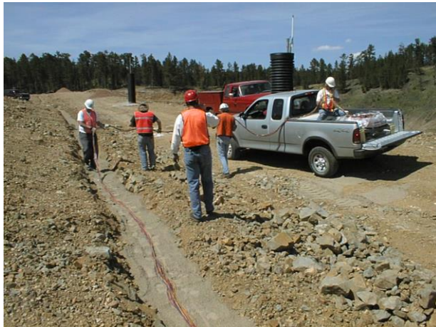
Figure 13. BurRec fabricated and installed 52-miles of wire for the electrode-arrays.
