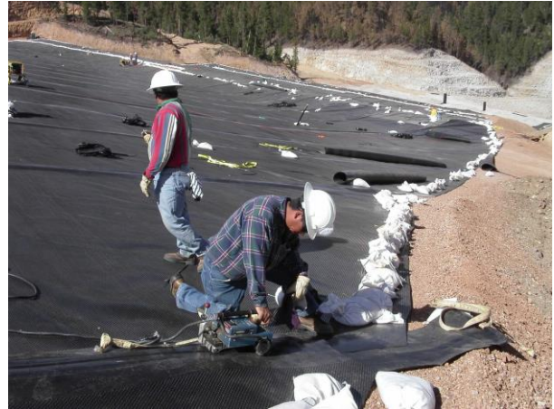
Figure 7. Lay-down and seaming of low-linear density polyethylene liner.
