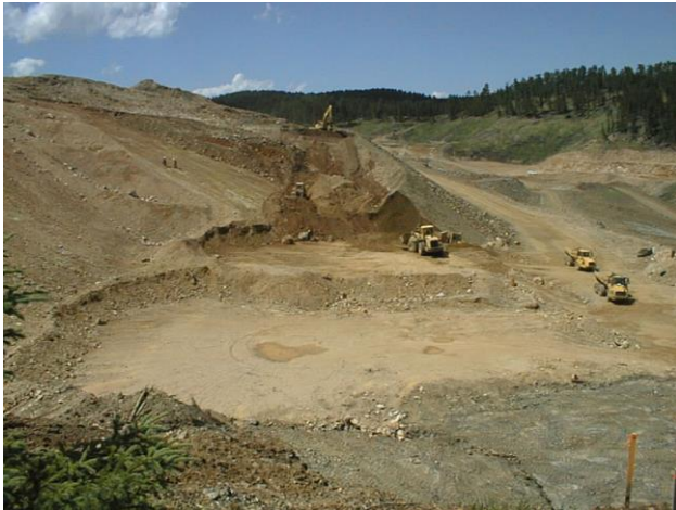
Figure 3. Hauling and reshaping valley fill.
