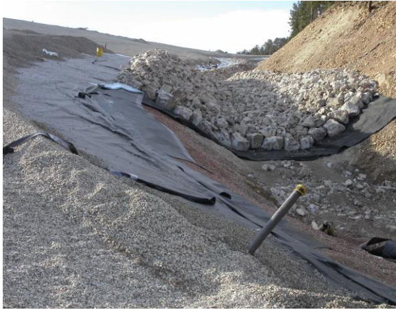
Figure 6. Diversion bentonite bedding, geo-composite liner, and riprap
