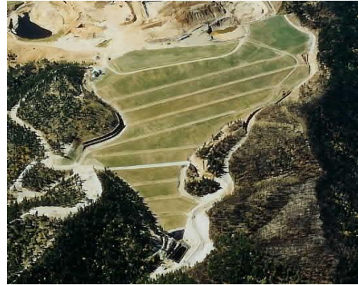
Figure11. Fall 2003 view (facing west) of the capped repository; five lower slope-segments and benches drain to diversions at right, bypassing ARD impoundment and exiting out lower Ruby Gulch; five upper slope-segments and benches drain to diversions at left, exiting into adjacent drainage to the south .
