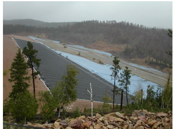
Figure 5. Geomembrane laid and drain-rock placement on slopes and benches.
