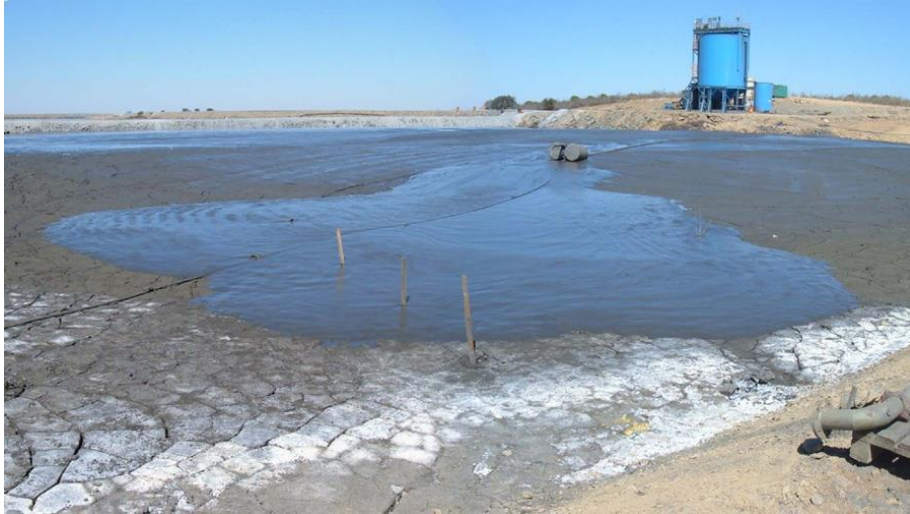
Figure 11. Overview of paste plant and pilot cell.
