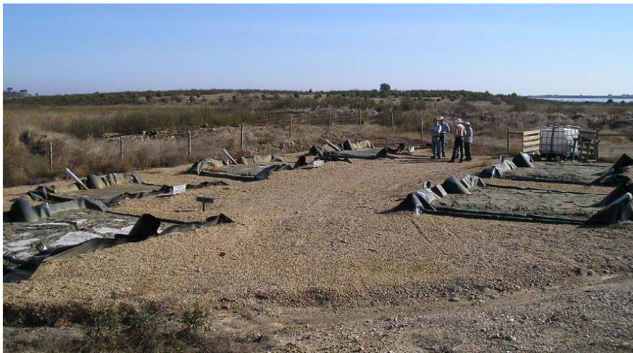
Figure 3. Overview of completed cells.
