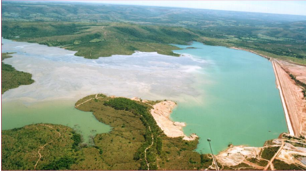
Figure 5: Tailings dam facility
